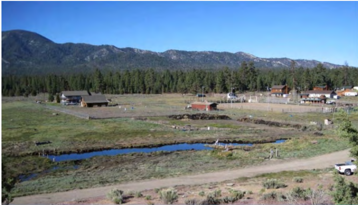
Photo 3-2. Shay Pond After Dredging
