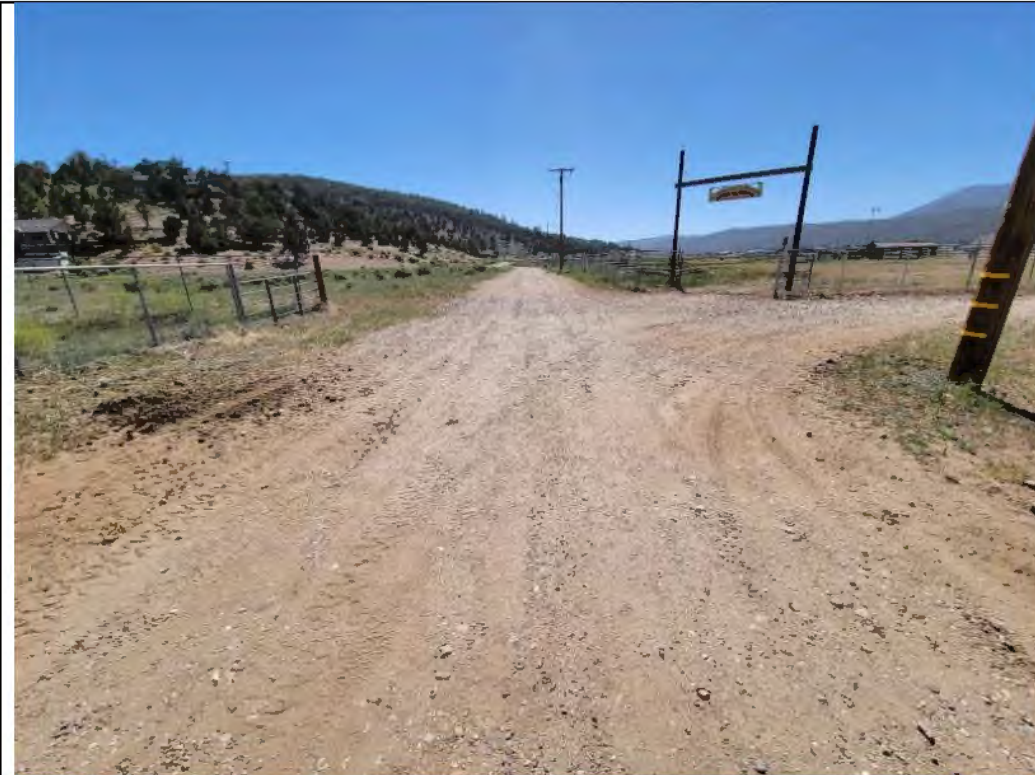
Photo 19. New 4-inch Shay Pond conveyance pipeline alignment in Cascade Street; looking east from west end of alignment (2022).
