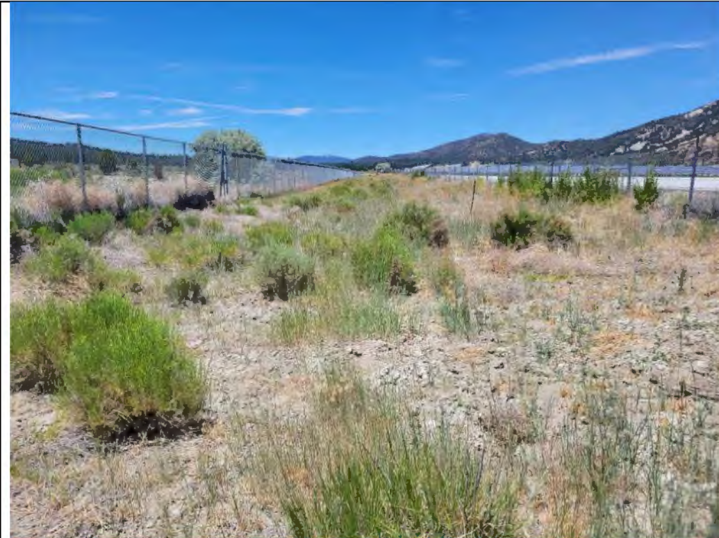
Photo 5. Baldwin Lake conveyance pipeline alternative; looking west along alignment from the east end of the alignment within the BBARWA WWTP (2023).
