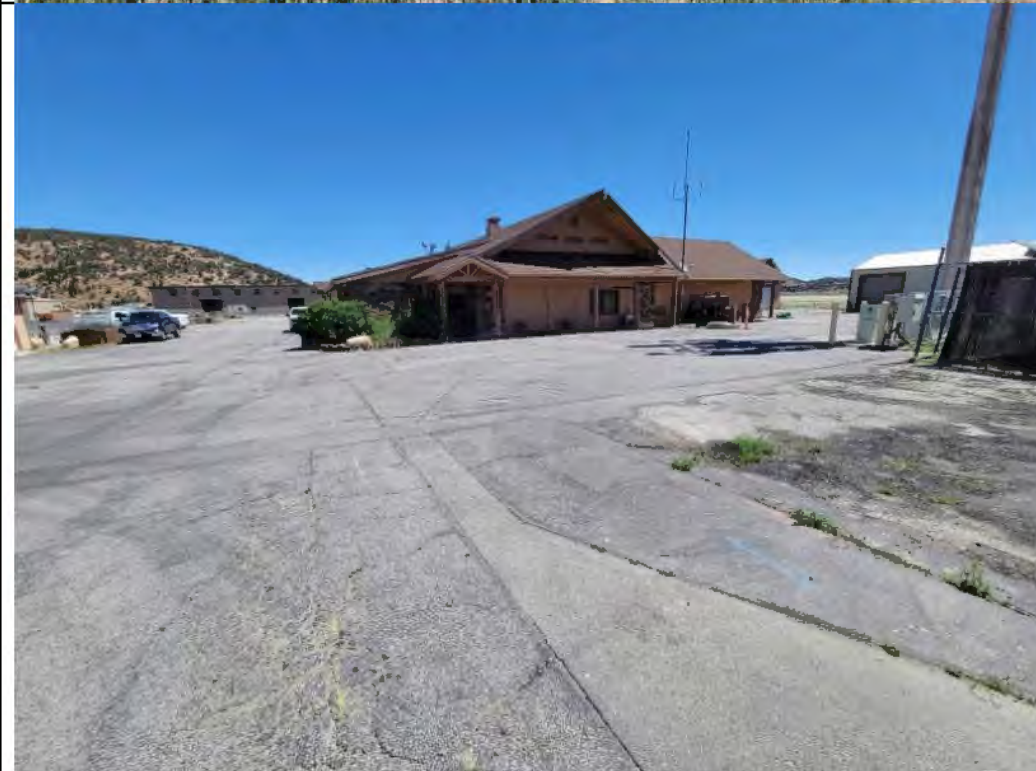
Photo 16. BBARWA WWTP Upgrades site (2022).
