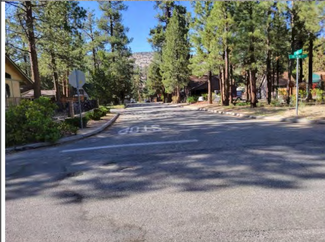
Photo 2. Representative photo of the East Neighborhoods conveyance pipeline alternative; looking north along Pintail Drive from the intersection of Pintail Drive and E Mountain View Boulevard (2022).
