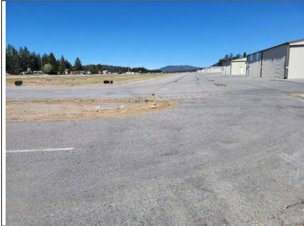
Photo 11. Representative photo of the North Airport Corridor conveyance pipeline alternative; looking west along the airport taxiway (2022).
