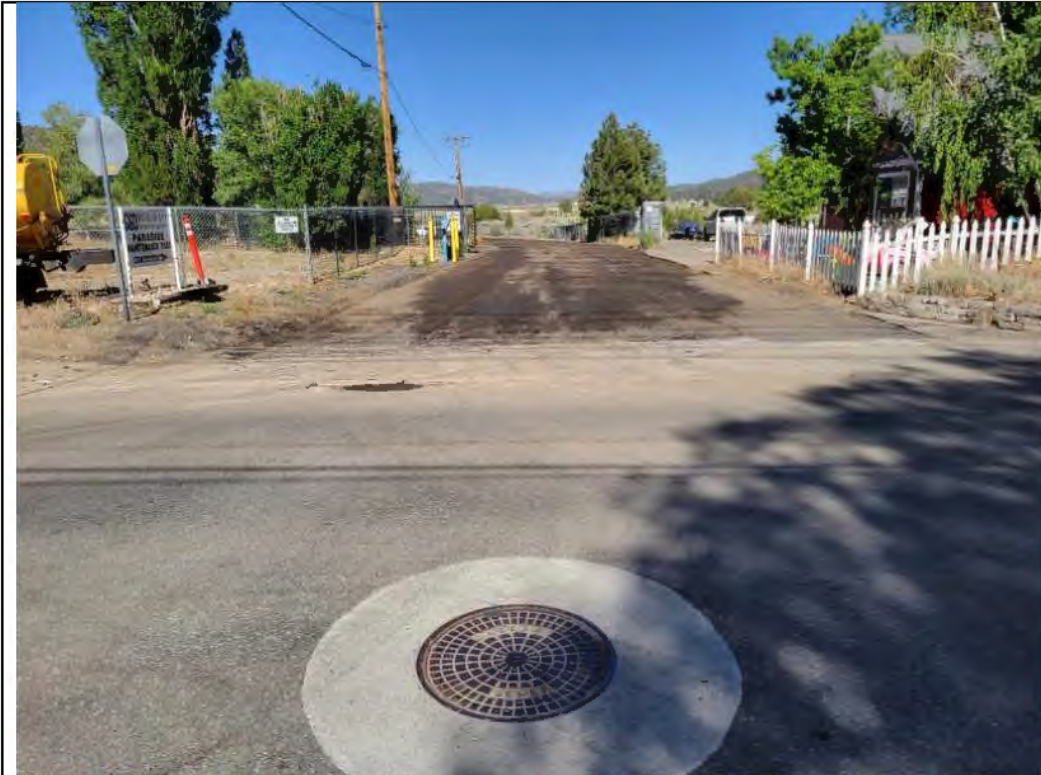
Photo 9. Baldwin Lake conveyance pipeline alternative; looking east along alignment from the west end of the alignment at Paradise Way (2022).
