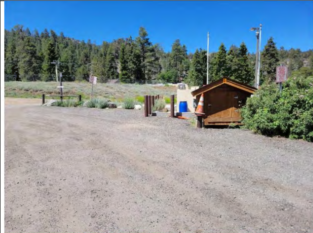
Photo 21. New Sand Canyon Recharge booster pump station site (2022).
