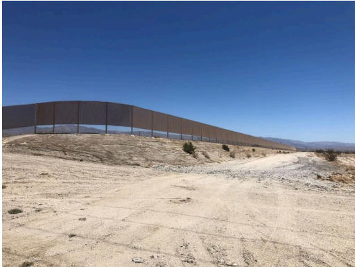
1. North Side of the property viewed from Rio del Sol Road
