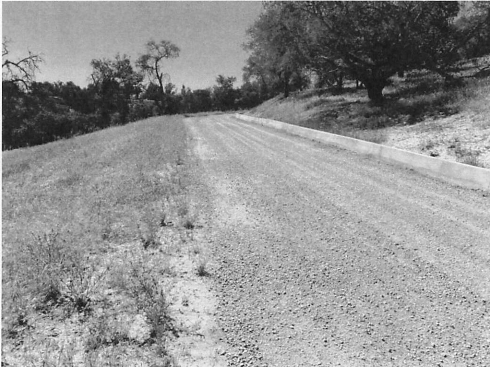
Photo 8. View of the existing driveway leading from Stage Springs Road to the old arena area proposed for development. Disturbed areas along the margin had been seeded with an erosion control seed mix of varying species.
