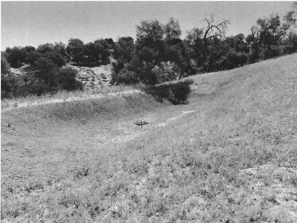
Photo 12. Stormwater basin constructed along the access road collects runoff from the driveway. There was no sign of past ponded water or hydrophytic vegetation and the entire area was mapped as ruderal due to disturbance.
