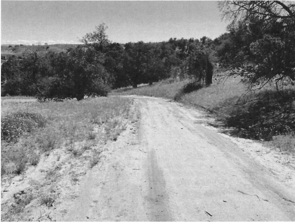
Photo 9. View of the access road upon its approach to the former arena. This section would be improved and have a concrete surface near the structures.
