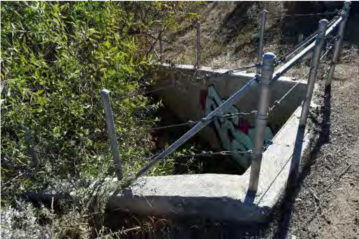
Photo Site 12 – Looking at riparian headwall
