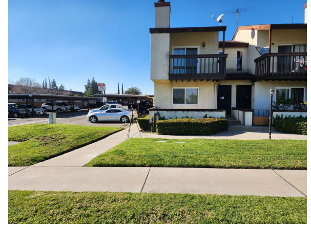
Figure 6: ST-6 9100 Acaia Ave
