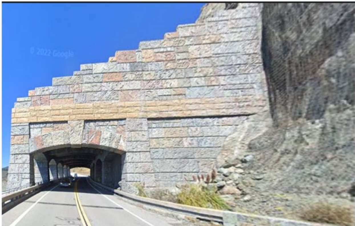
Rock Shed Example in California on the Big Sur Coast (05-Mon-1 PM 21.0).
