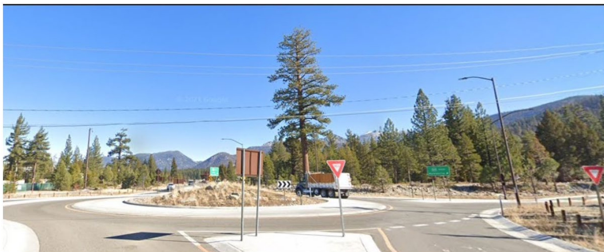
Example of roundabout in Lake Tahoe. Features include landscaping and colored concrete.
