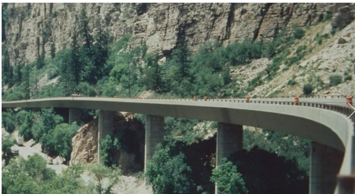
Viaduct examples on I-70 in Colorado. Colored concrete matches local rock. Vegetation around viaduct columns visually integrates structure. Bridge barrier architectural treatment is compatible with the adjacent bridges.
