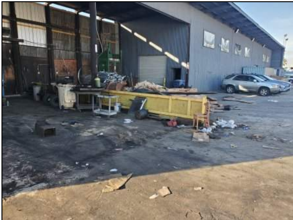
View of service/storage building at 825 E State St.
