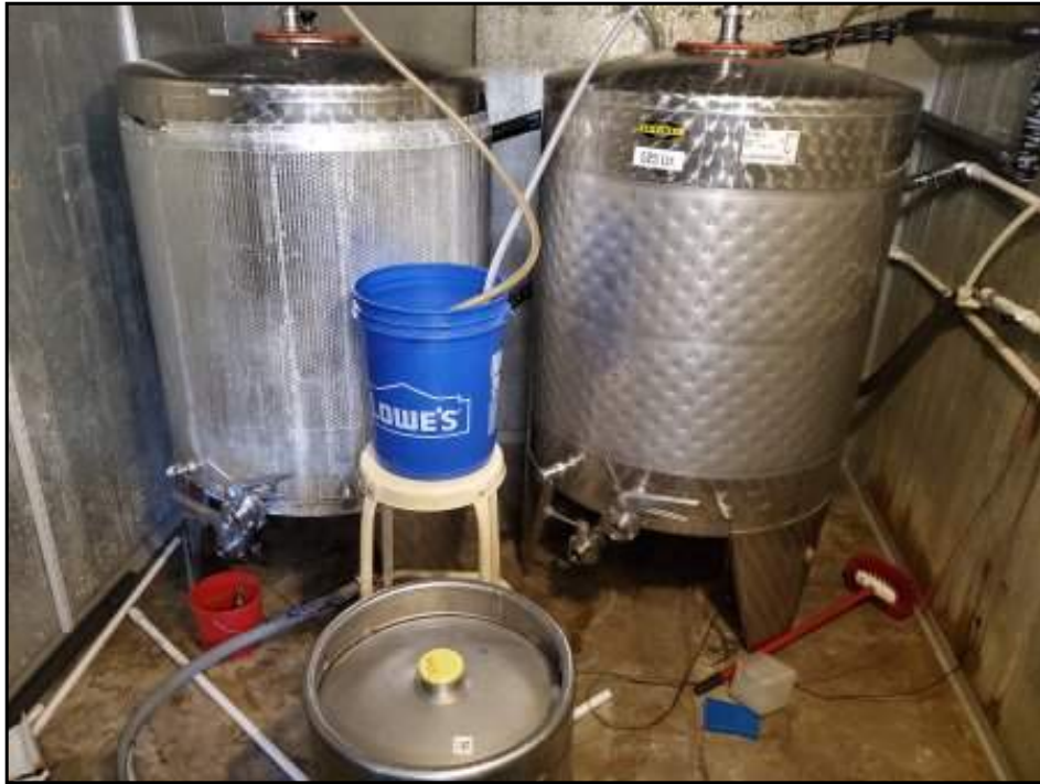
View of fermenting room at Strum Brewing.
