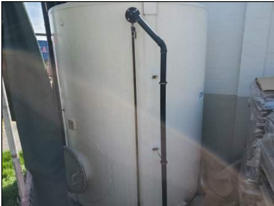
View of approximate 10,000-gallon empty AST labeled as storm water at northeast corner of warehouse building in western portion of Property.
