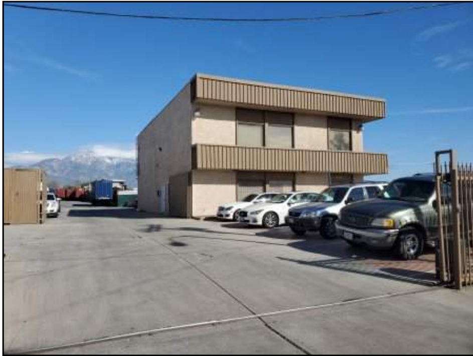
View of two-story commercial office building located at 807 E State Street.
