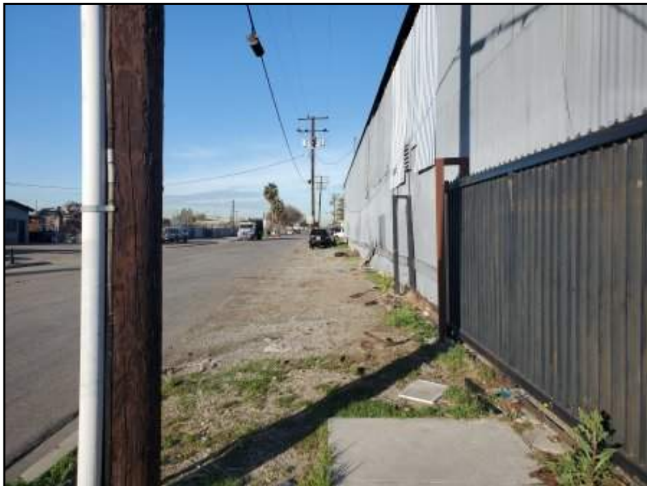
View of southern Property boundary (looking west).
