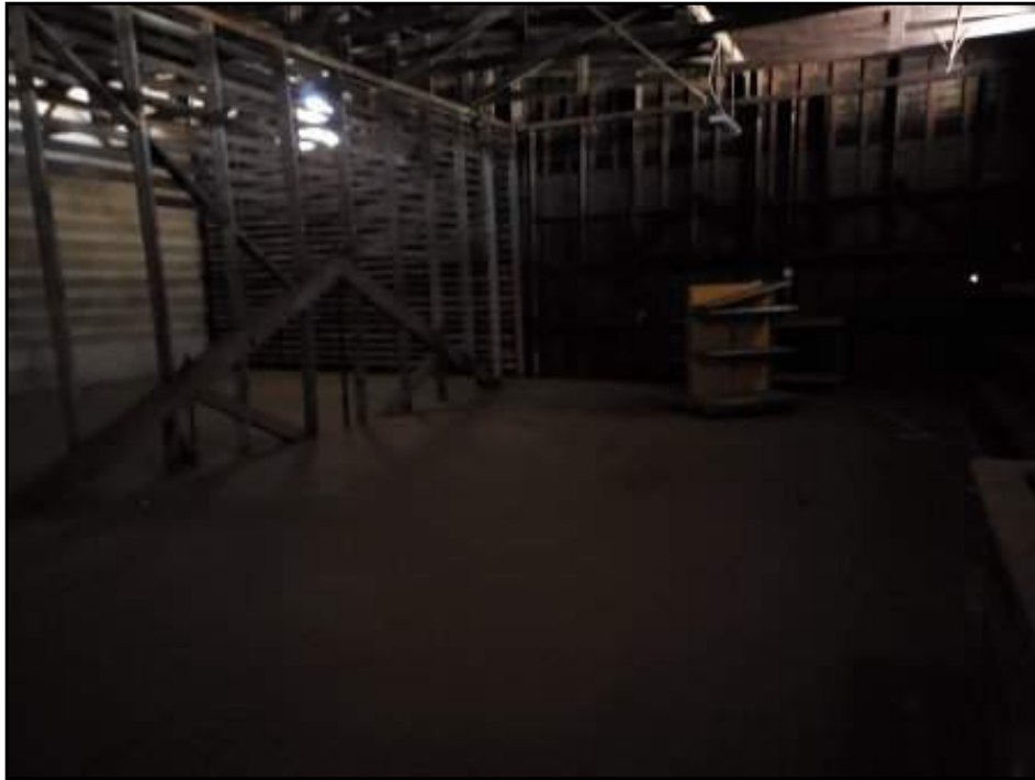
View of interior of second floor of vacant portion of 717 E state Street.
