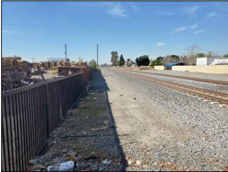
View of northern boundary of Property (looking west).
