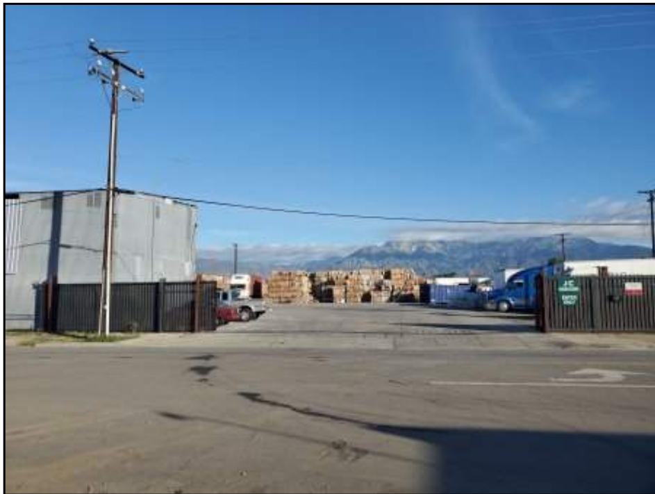
View of eastern portion of Property (825 E State Street/316 Bon View Avenue).
