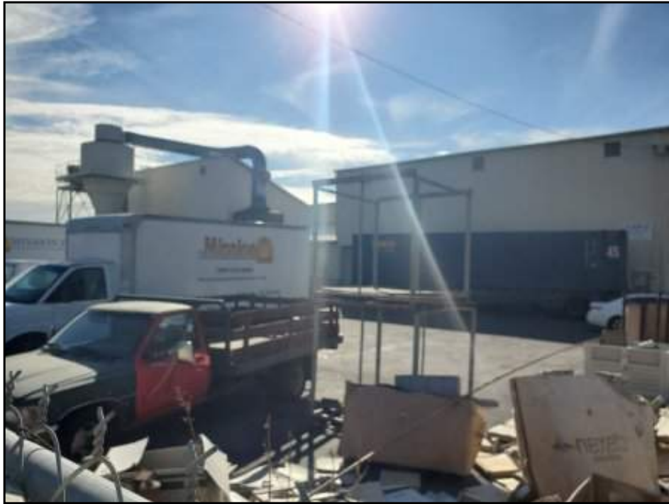
View of dust collection system on north side of warehouse buildings located in western portion of Property.
