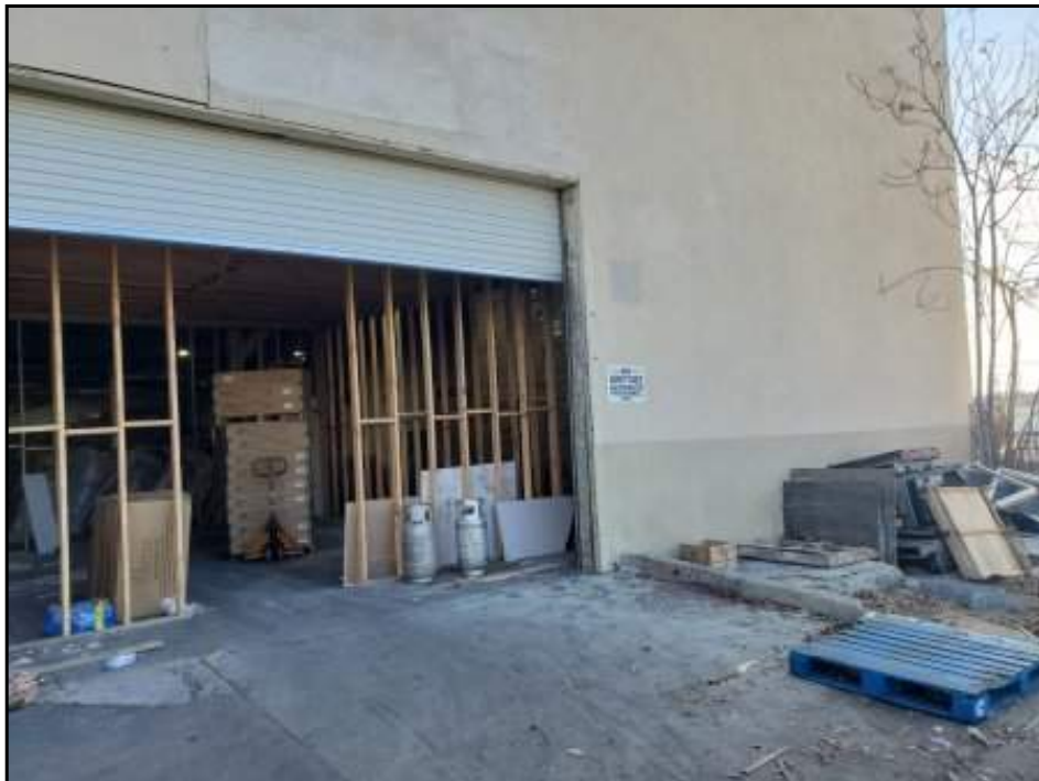
View of entrance to 717 E State Street.
