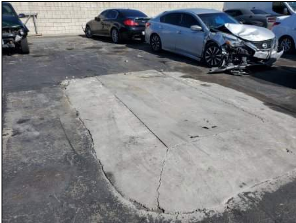
View of concrete patch area at 810 E Main Street tow yard.
