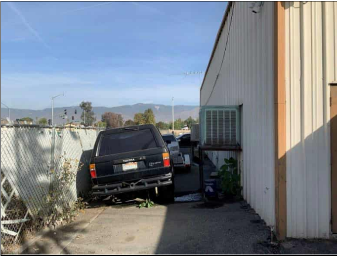
97. 97. Property 11, east side of the service building, view facing north.
