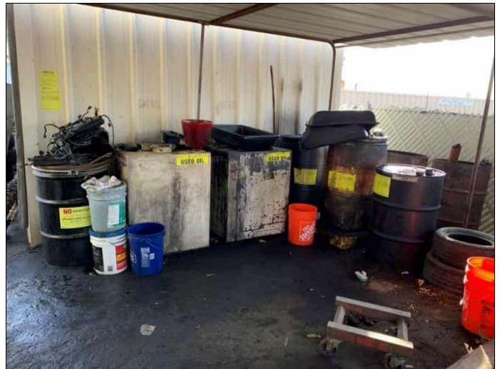
94. 94. Property 11, hazardous waste storage area located adjacent to the south side of service building, view facing southeast.
