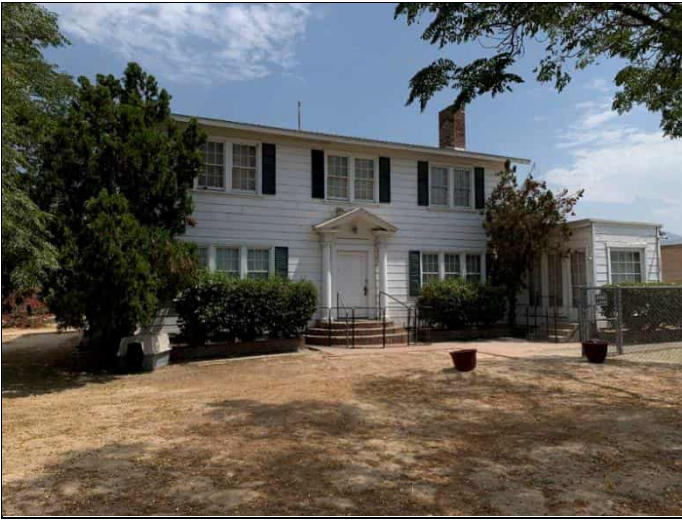
67. Property 9 residence/septic tank at 27136 3 rd Street (southeast corner of the property), view facing north.
