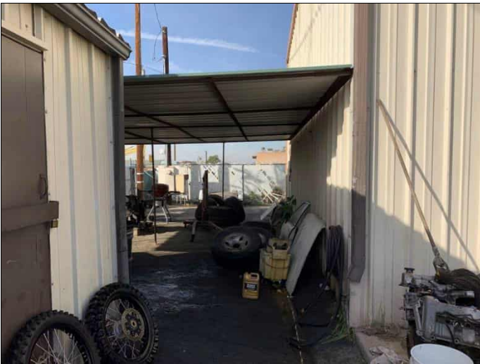
93. 93. Property 11, service building on the south side of property, view facing west.
