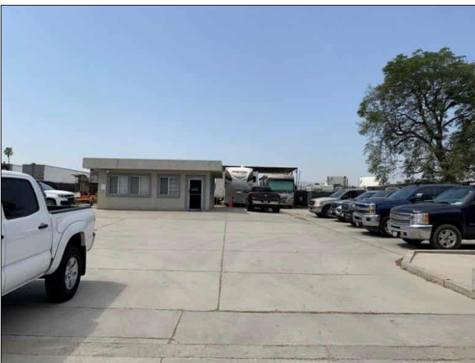
23. Property 4 Office parcel (off of 5 th Street) southern portion of the property, view facing south.
