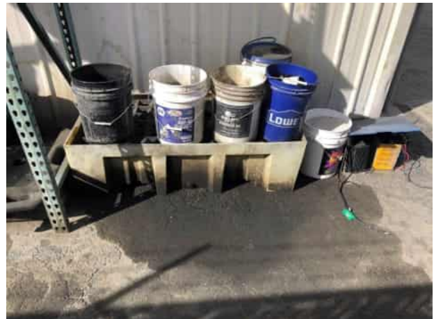
18. View of the de minimis staining on the asphalt.
