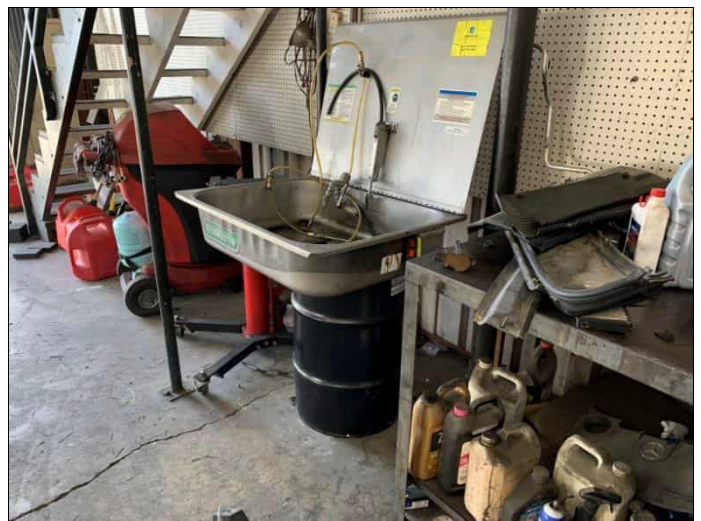
90. 90. Property 11, parts washer on the south side of the service building, view facing east.
