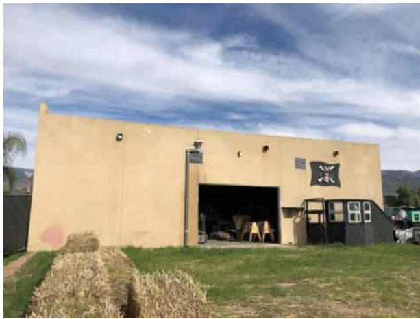
3.View of the subject property building from the south.
