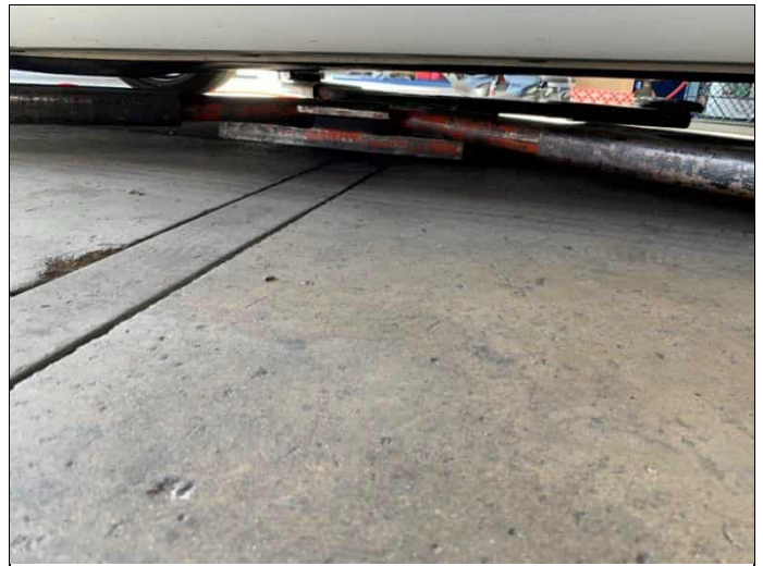
88. 88. Property 11, one of the two in-ground hydraulic lifts, view facing south.
