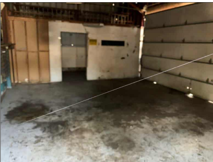
59. Property 7 former auto repair facility building interior, view facing south.
