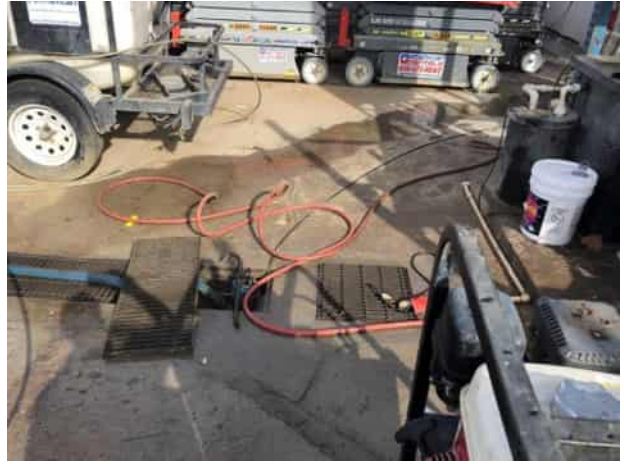
8.View of the trenched mud-pit where rental equipment is hosed off.
