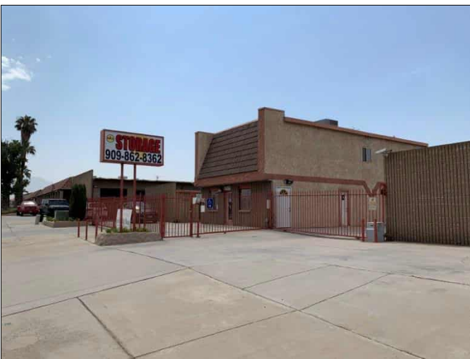
77. Adjacent properties to the east, view facing southeast.
