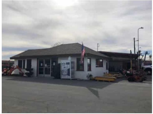
2.View of the main office building on the north.
