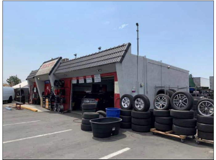
62. Property 8 building on the southern portion of the facility, view facing southeast.
