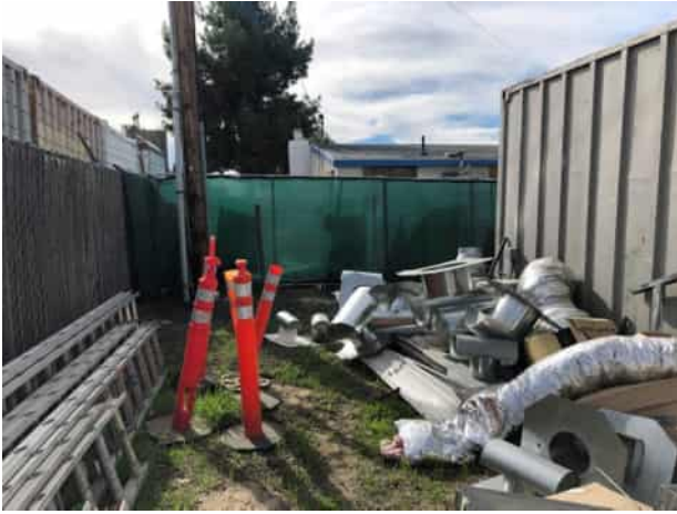
13. View of stored ducting materials on the south-east.
