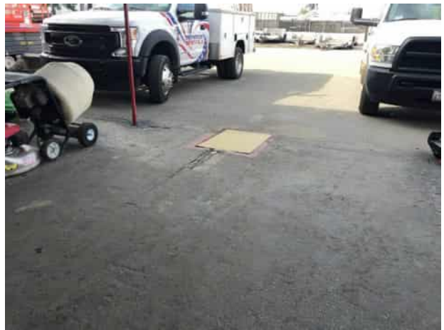
10.View of the stormwater drain collection area.
