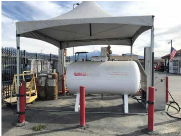
5.View of the propane tank on the north of the property.
