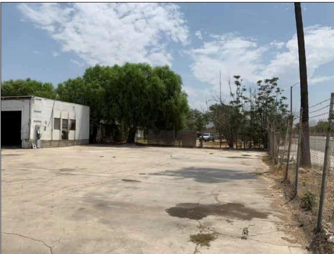
57. Property 7 former auto repair facility from the southwest corner of the facility, view facing east.
