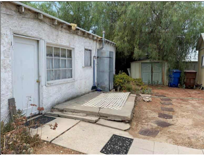
69. Property 9 residence/septic tank at 27132 3 rd Street (southwest corner of the property), view facing west.
