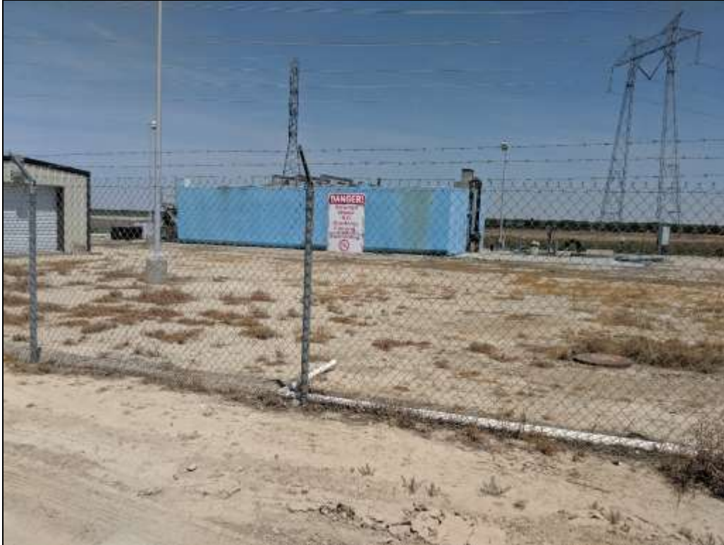
Photo 1. Typical site existing conditions of the fenced in treatment plant site.
