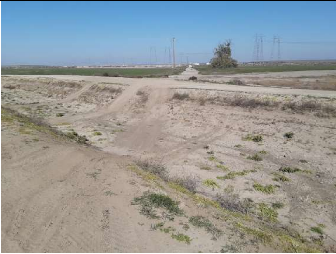
Photo 9. Looking N along proposed Water and Sewer Connection Pipeline alignment from S side of Buena Vista Water Storage District canal.
