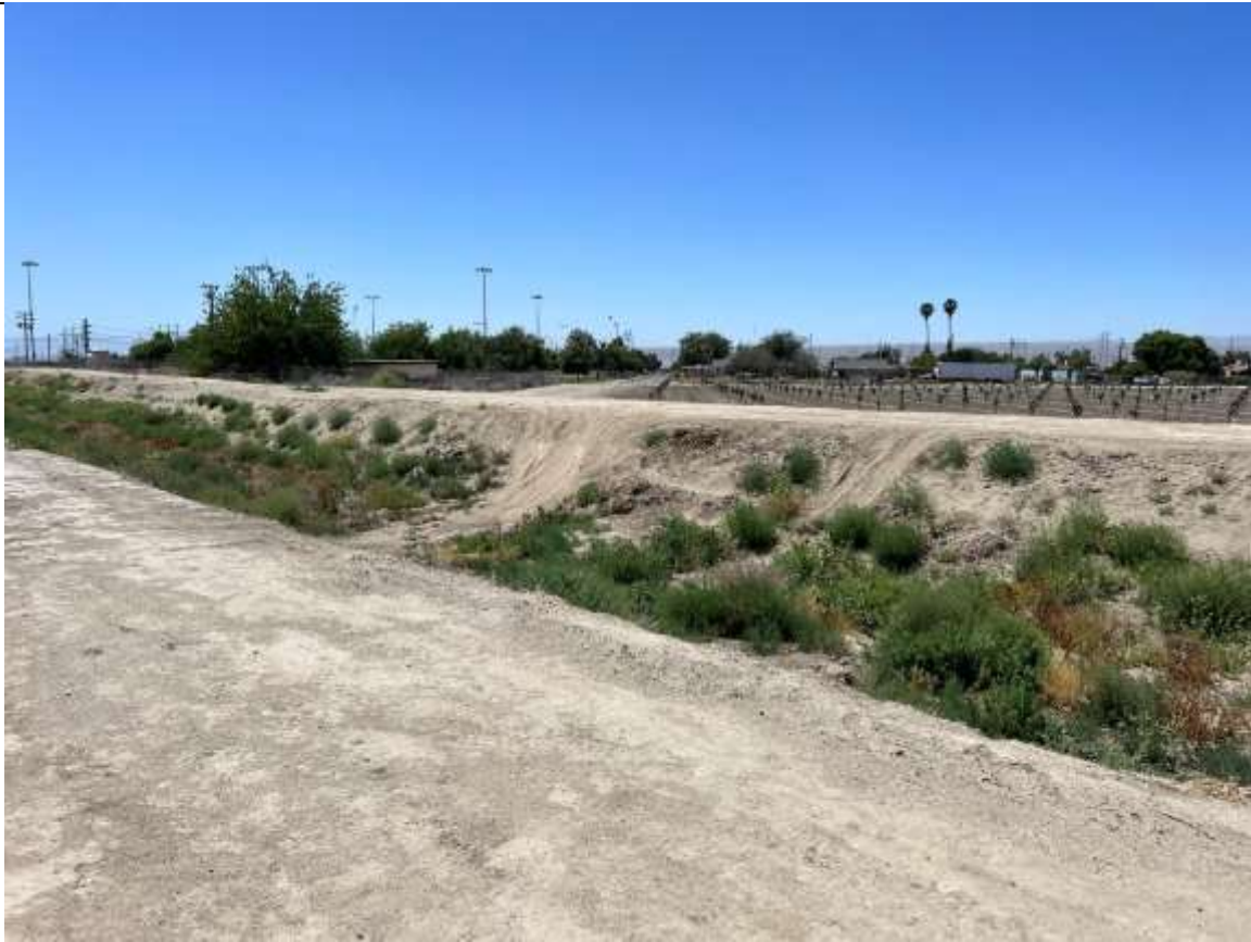
Photo 8. Looking S along proposed Water and Sewer Connection Pipeline alignment from N side of Buena Vista Water Storage District canal.
