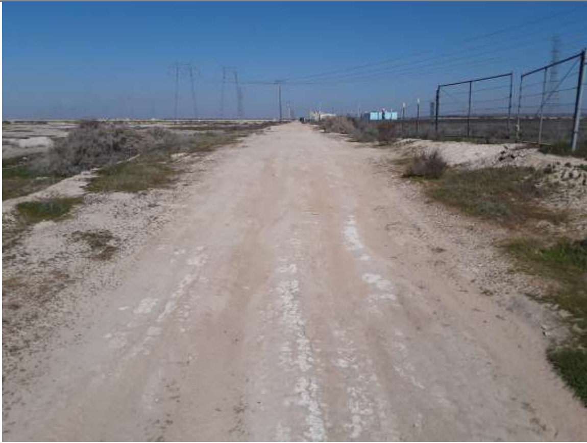
Photo 5. Looking N along access road between existing WWTP (right) and adjacent parcel S of the proposed Solar Field Site from N end of the proposed Water and Sewer Connection Pipeline alignment.
