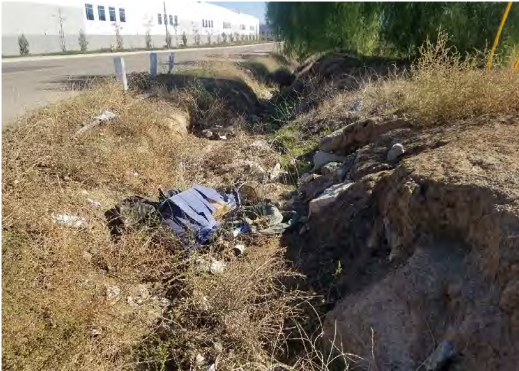
Photograph 5: View depicting western terminus of roadside ditch, immediately south of Rider Street.
