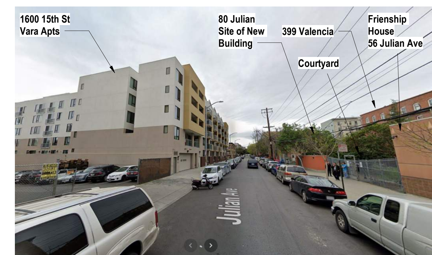
D) Julian Ave - Facing Side
