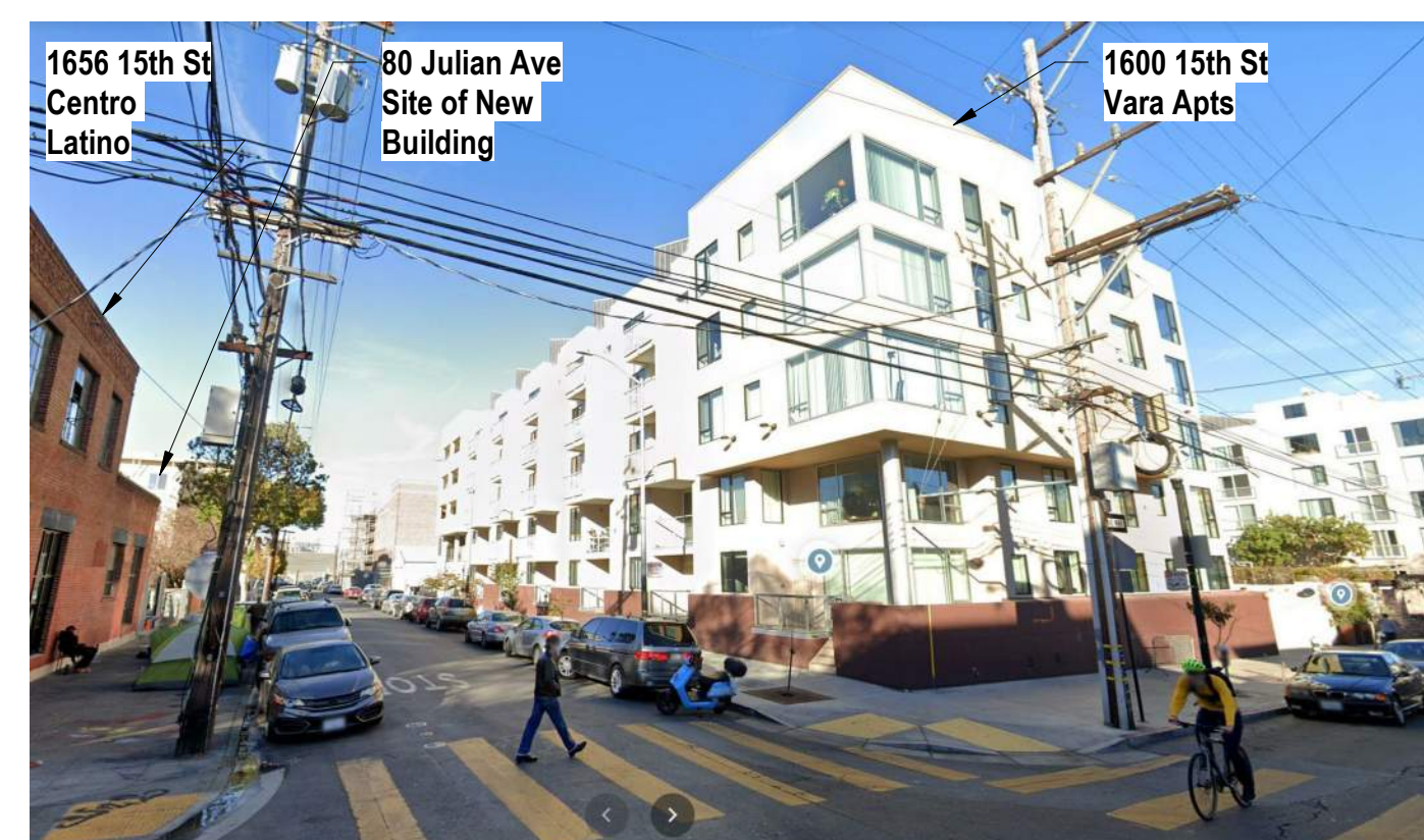
A) Julian Ave - Facing Side
