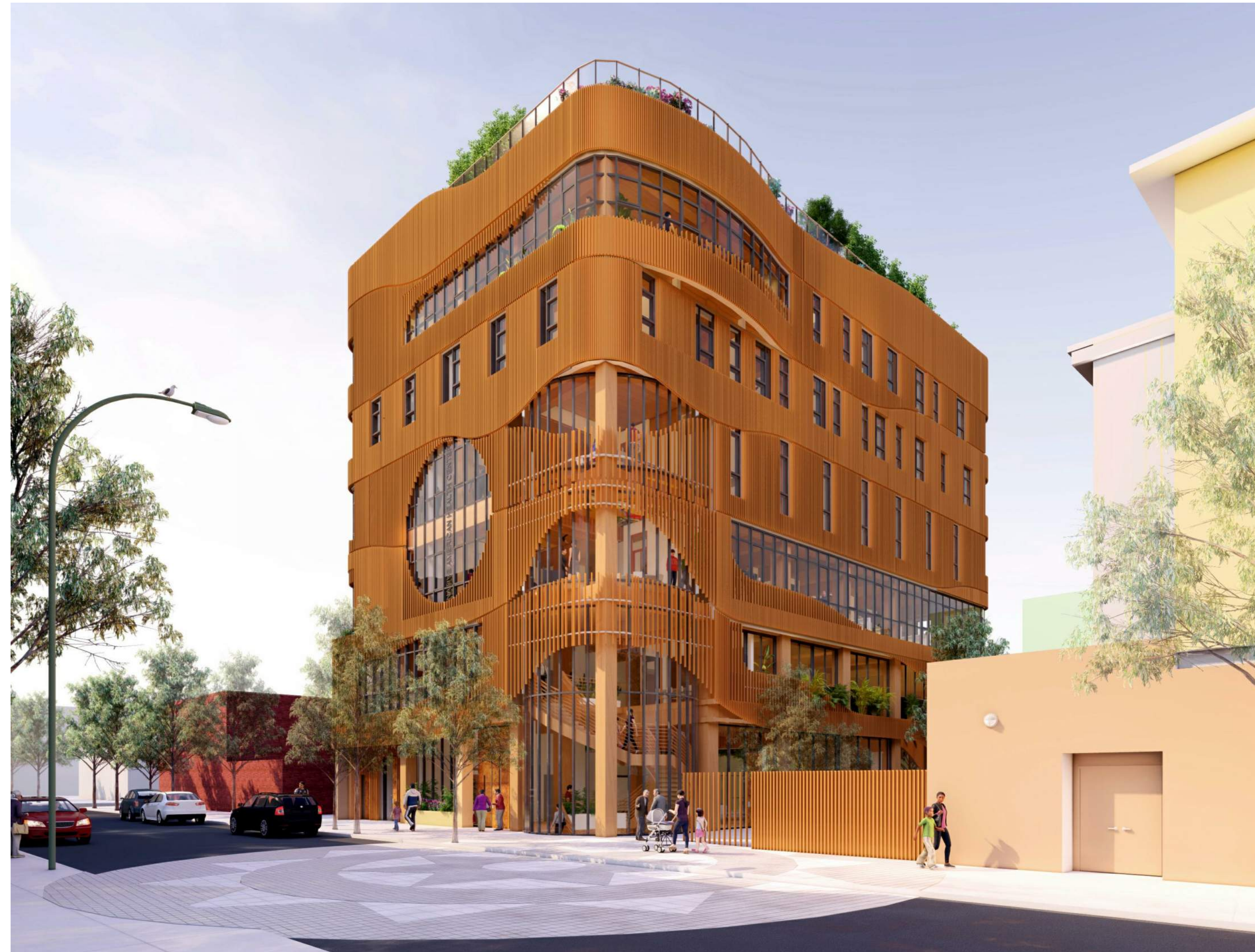
VIEW FROM JULIAN AVE. LOOKING TO SOUTH WEST
