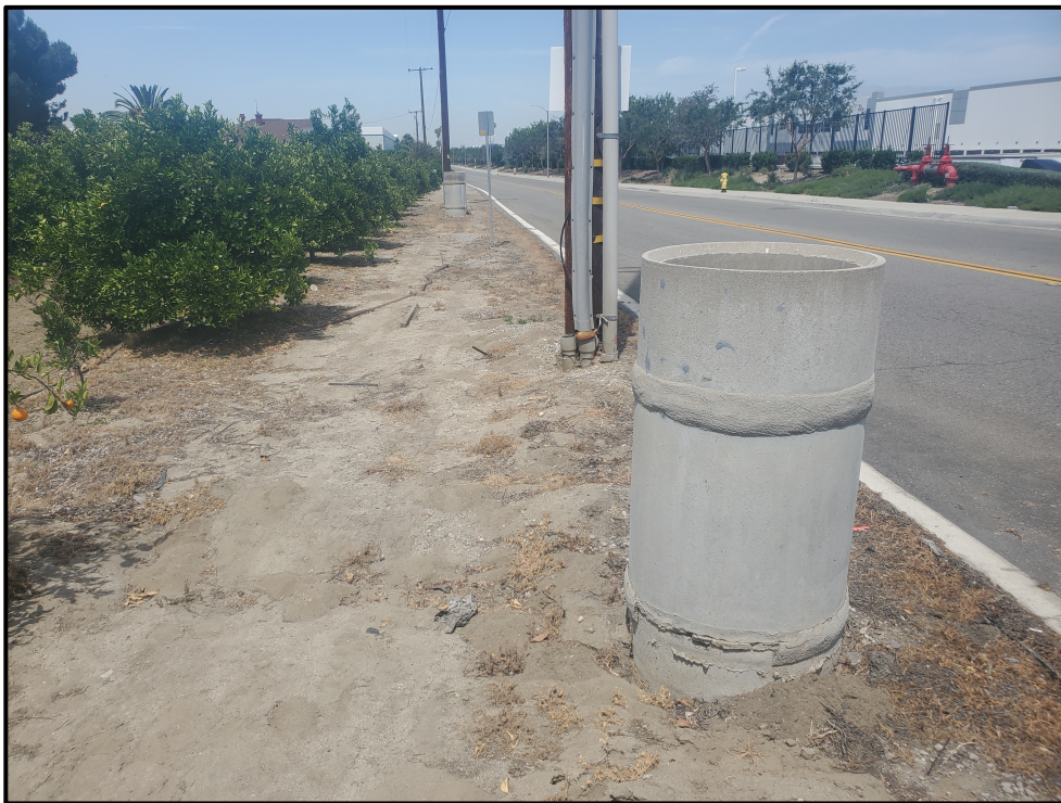
Plate 3.2–4: View of the newly identified irrigation features associated with Site P-36-024296, facing south.
