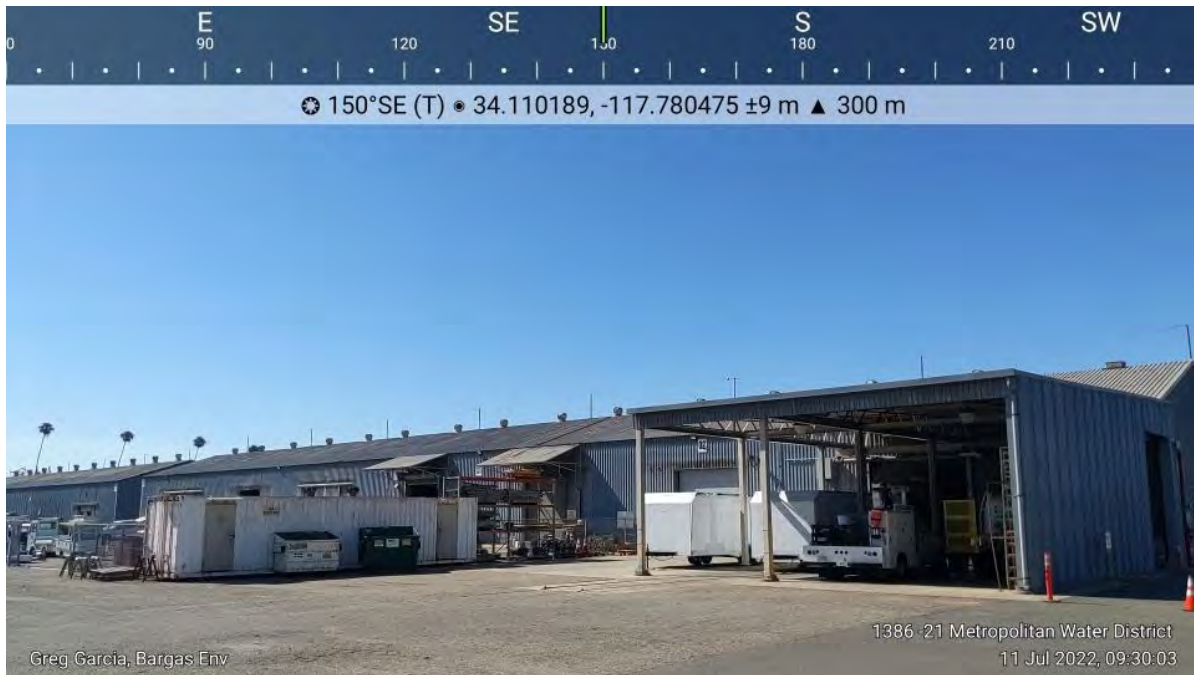
Photo 9. Representative photo of the La Verne Warehouse Facilities proposed for demolition and replacement with new warehouse facilities. Photo looking southeast from inside the Plant.
