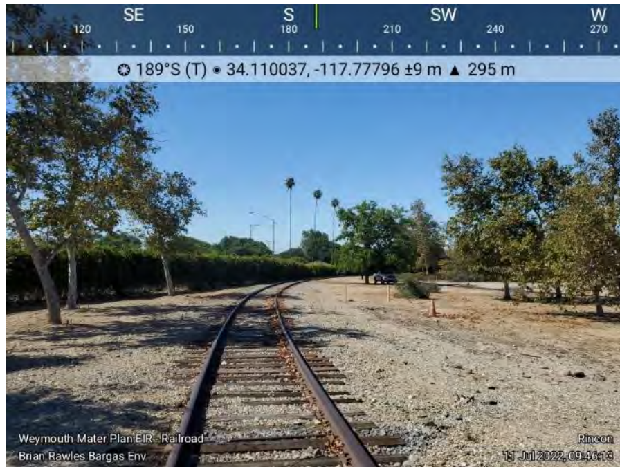
Photo 5. Representative photo of a section of the Water Treatment Chemical Delivery Railroad Tracks proposed for replacement within the Weymouth Plant. Photo looking southward from inside the Plant.
