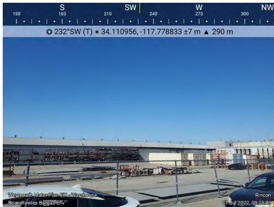
Photo 8. Representative photo of the La Verne Warehouse Facilities proposed for demolition and replacement with new warehouse facilities. Photo looking southwest from inside the Plant.
