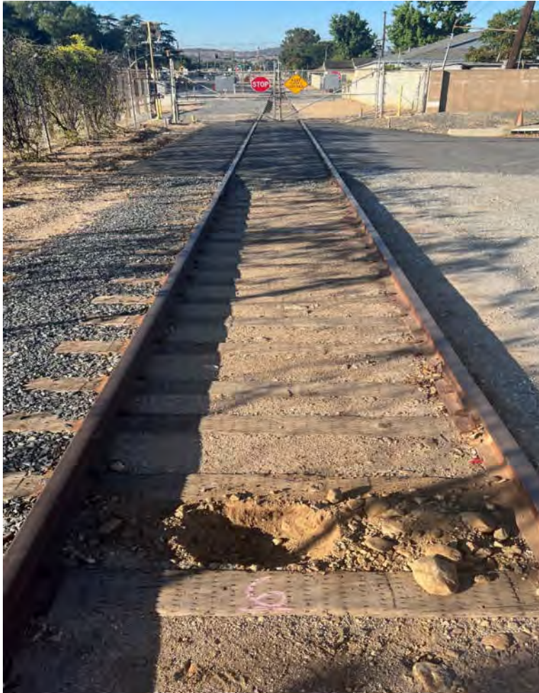
Photograph 1. Example of a single sampling location along the water treatment chemical delivery railroad tracks. Soil was sampled at the mid-point between railroad ties.
