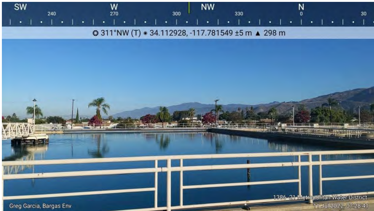
Photo 7. Representative photo of one of two basins proposed for rehabilitation. Photo looking northwest from inside the Plant.
