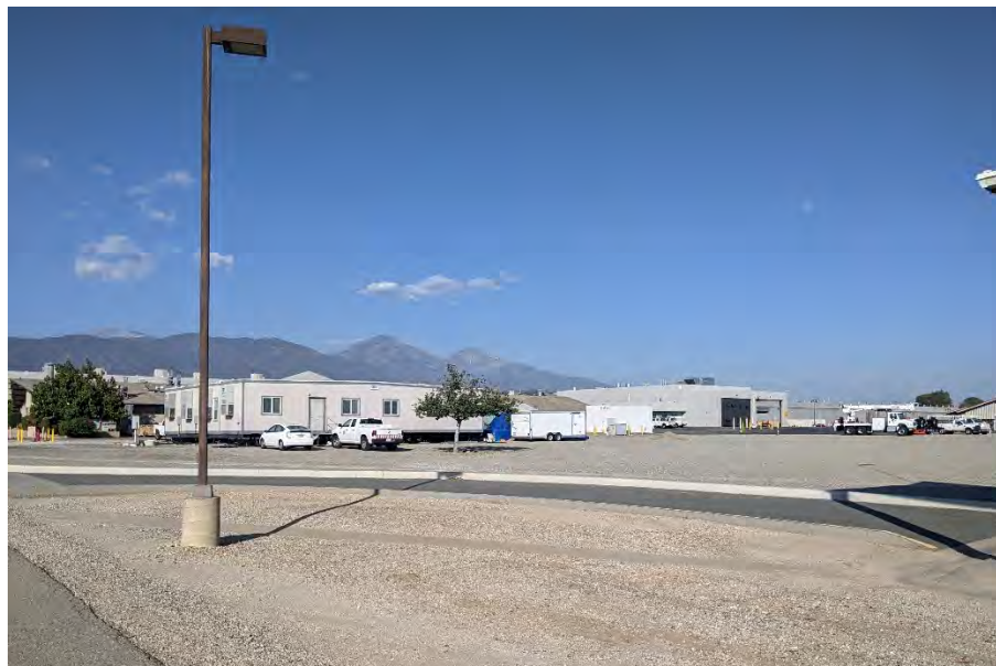
Photo 10. Representative photo of the new proposed location of the New Field Engineering Building. Photo looking northward from inside the Plant.
