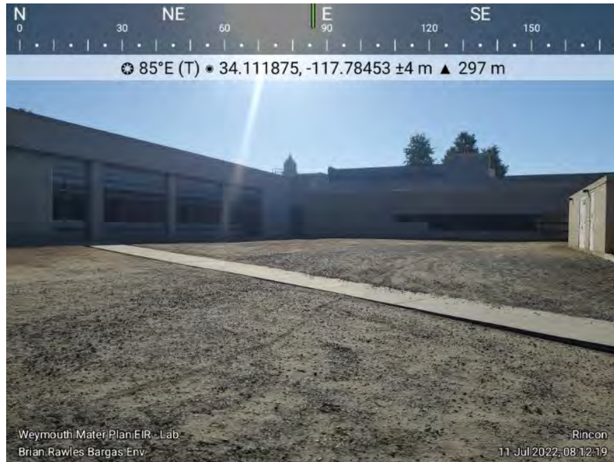
Photo 1. Representative photo of the Water Quality Laboratory Building (west-facing building) proposed to undergo various building improvements. Photo looking east from Sedalia Avenue.
