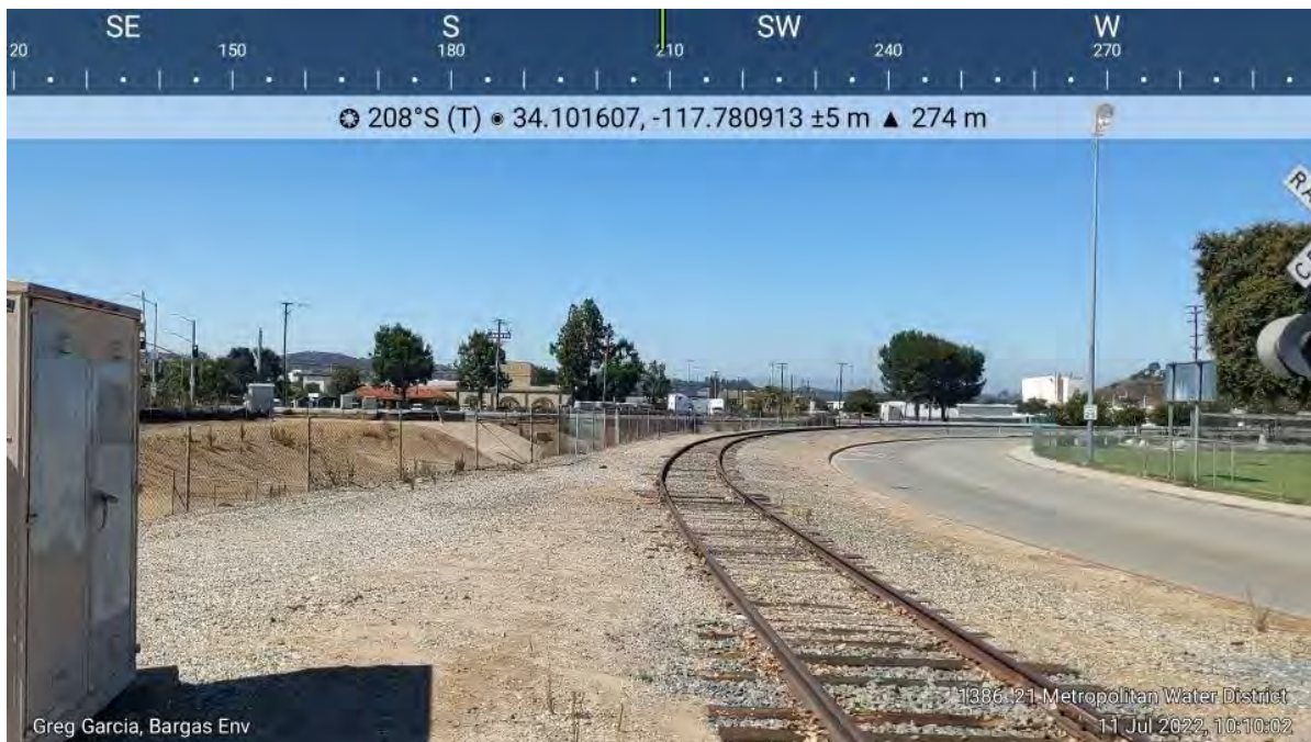
Photo 6. Representative photo of a section of the Water Treatment Chemical Delivery Railroad Tracks. This portion of the railroad tracks is located off-site of the Weymouth Plant and adjacent, but outside of, a Los Angeles County Flood Control District channel. Photo looking southwest along Palomares Avenue.
