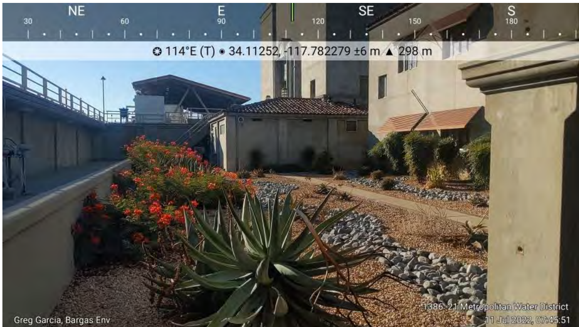
Photo 4. Representative photo of the Administration and Control Building (north-facing building) proposed to undergo various building improvements. Photo looking southeast from inside the Plant.
