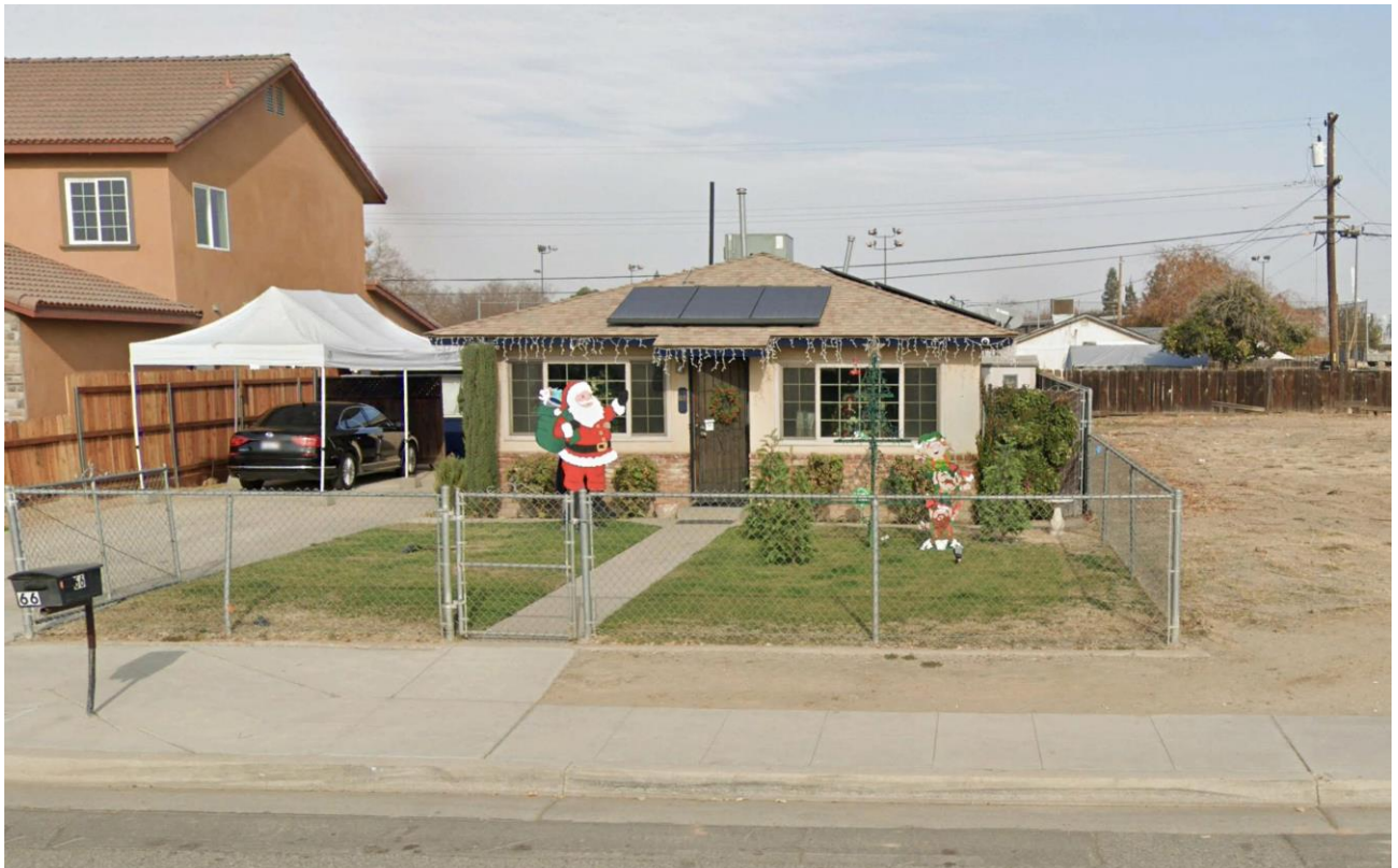
B) View looking north of the south facing façades of the garage (left), residence. 2/28/22. Acc. 2022IMG2crop
