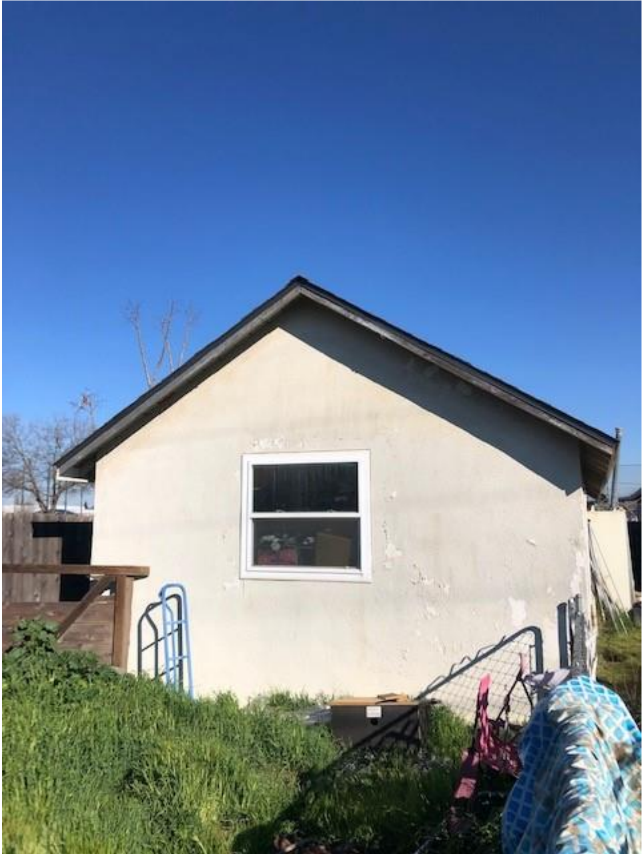
G) View looking north of the south facing façade of the detached garage. 2/28/22. Acc. #2022IMG5827
