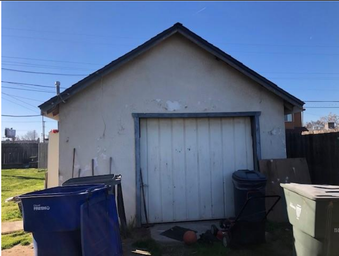
E) View looking south of the north facing façade of the detached garage. 2/28/22. Acc. #2022IMG5824
