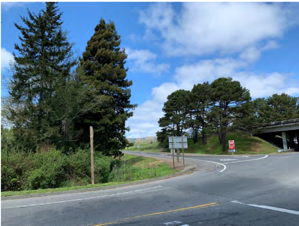
Photo 3. The western side of the Kenmar Road Interchange.
