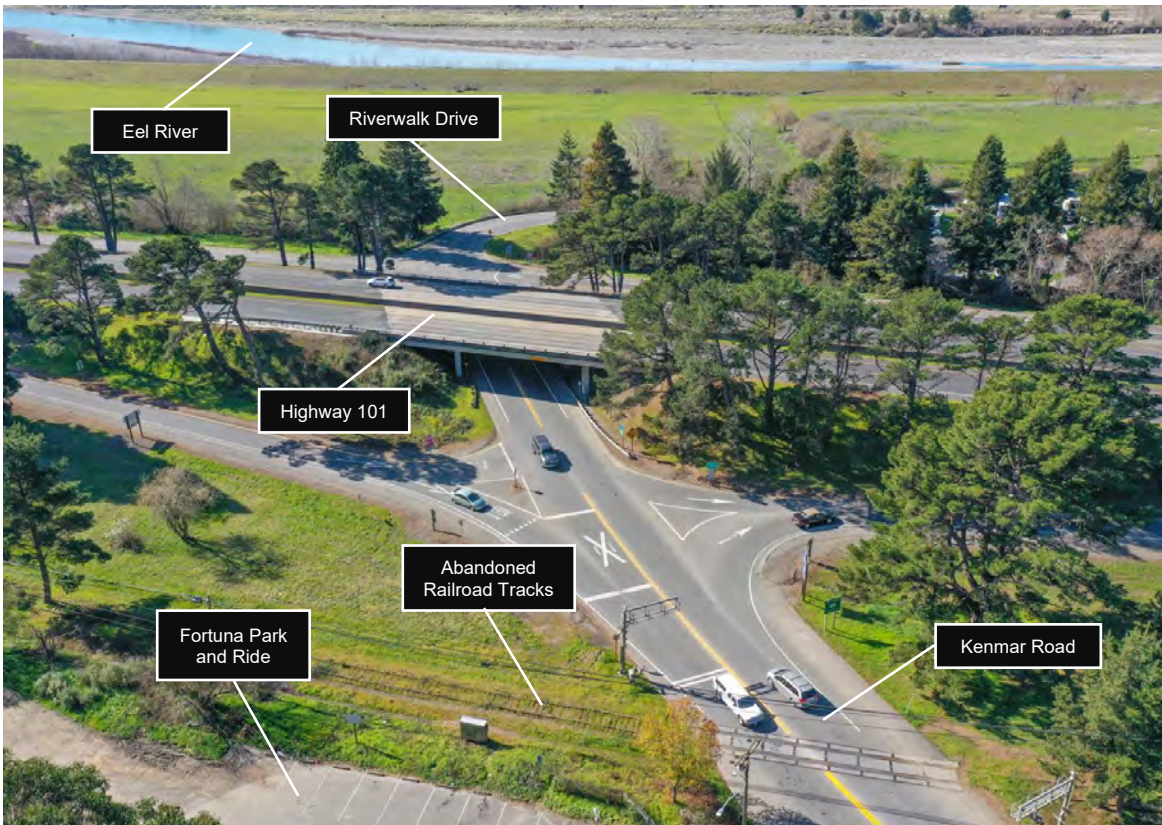
Exhibit 2 – Aerial view of the Project area looking west from the eastern portion of the Project area. Views of the Eel River to the west and abandoned railroad tracks and Fortuna Park and Ride to the east of the Project area.
