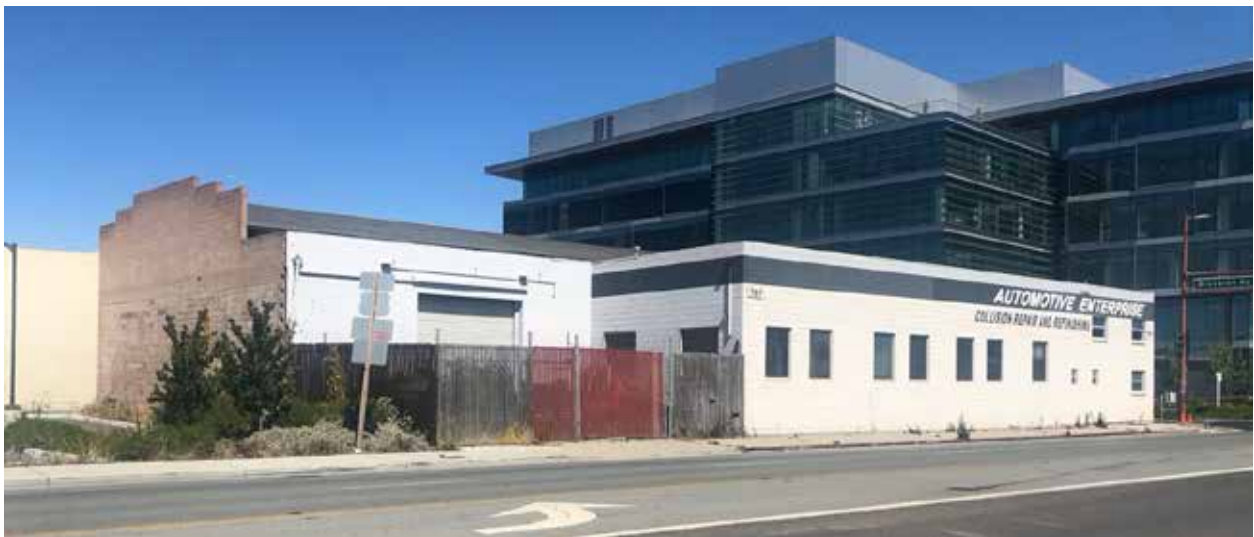
Fig.10 – 797 Industrial Rd. – Rear (northwest) and southwest side, from Industrial Rd.
