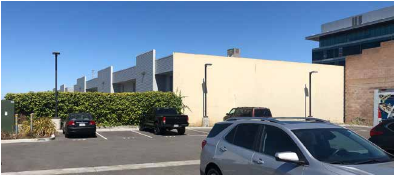
Fig.13 – 814-838 & 840-870 Bransten Rd. – Rear and southwest side, from Industrial Rd.
