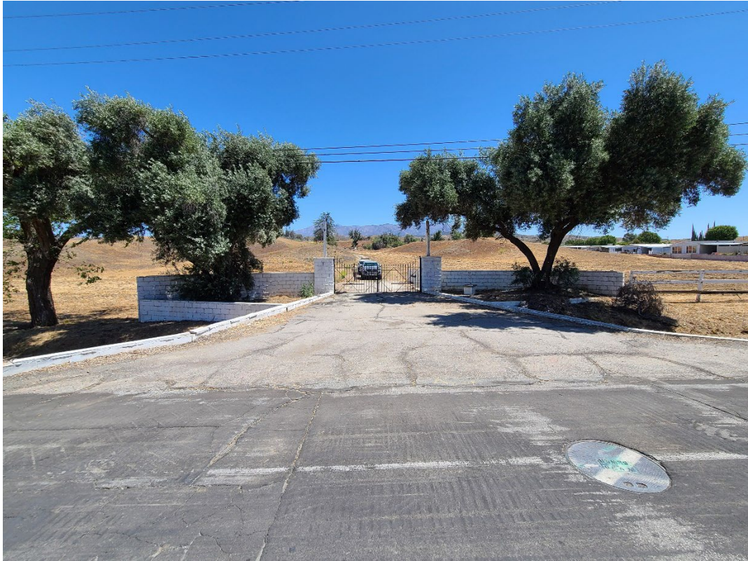
Figure 6-13. Cinderblock fence and gate (Feature 8) off Calimesa Boulevard, facing east.
