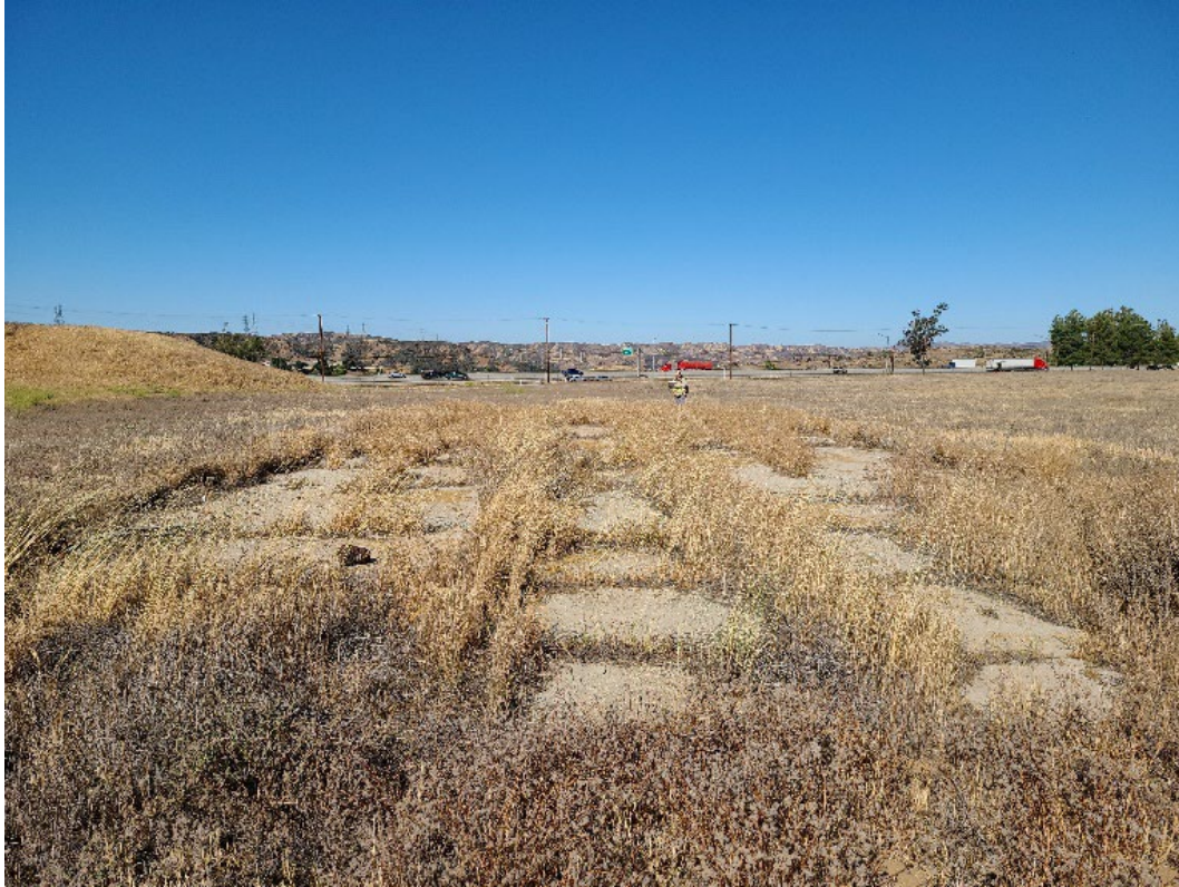
Figure 6-10. Overview of concrete slab foundation (Feature 3), facing southwest.
