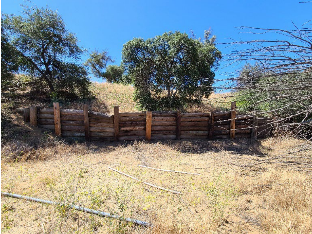
Figure 6-12. Overview of Feature 2, retaining wall, facing southeast.
