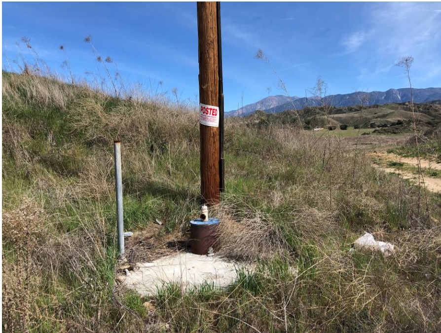
View of a metal riser pipe potentially associated with a water well observed on the Diocese of San Bernardino Property next to a power pole near where structures were formerly present.
