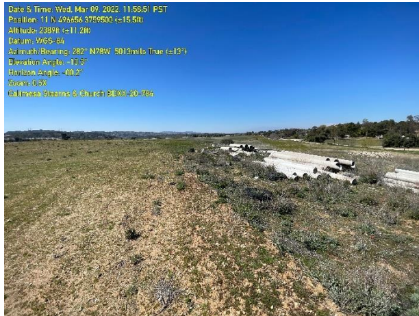
Piles of debris and old pipes (on right), northeast corner of site facing west (03.09.2022).
