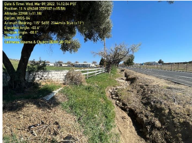
Roadside ditch along Calimesa Boulevard at southern corner of site, facing east-southeast (03.09.2022).
