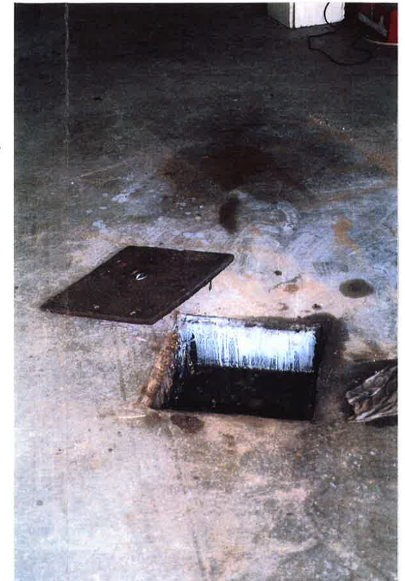
Drainage collection area located in the floor of the shop barn.
