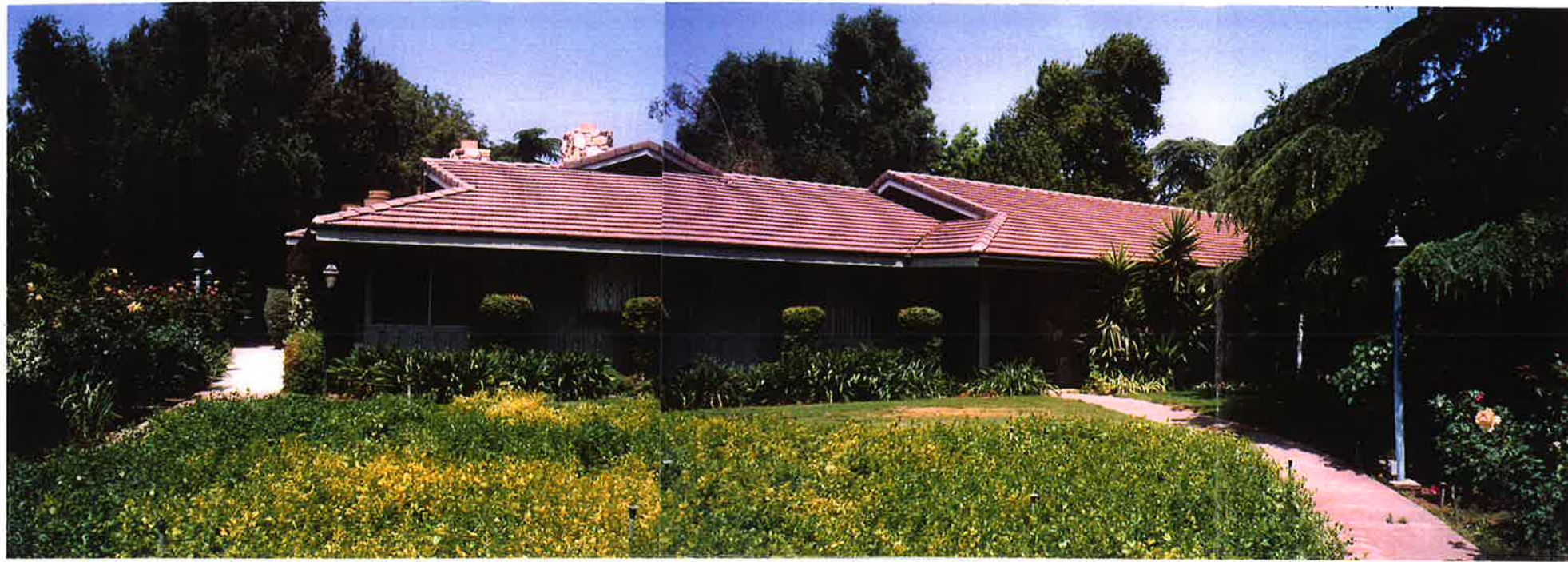
Main residence located at the Suzy Q Ranch.
