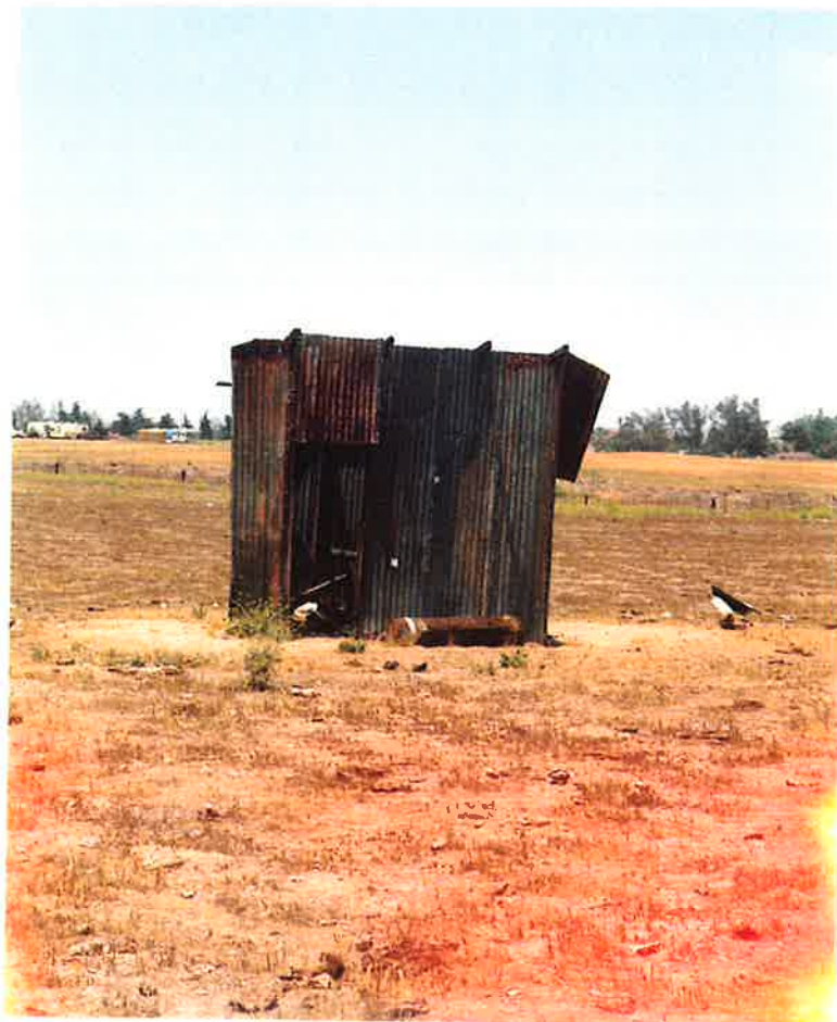
Inactive well located on-site
