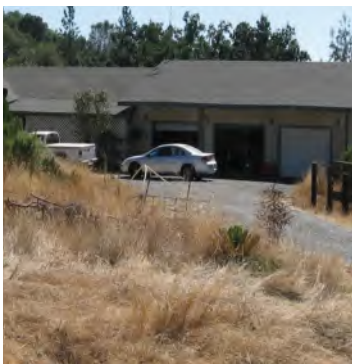
DEFENSIBLE SPACE NONCOMPLIANT
