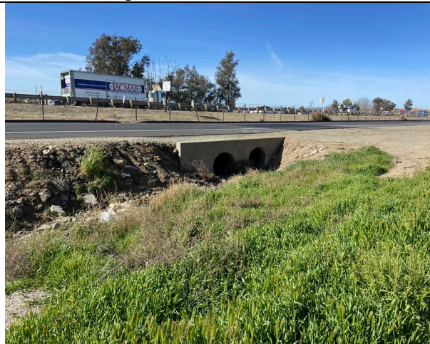
View of the concrete double-pipe culvert beneath Calimesa Boulevard.
