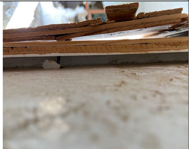
View of one of the crevices suitable for use by roosting bats created by the plywood nailed over the windows of the abandoned residence.
