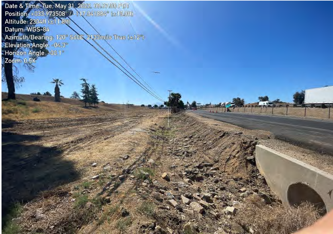
Manmade ditch (D3) facing southeast leading to under road crossing.
