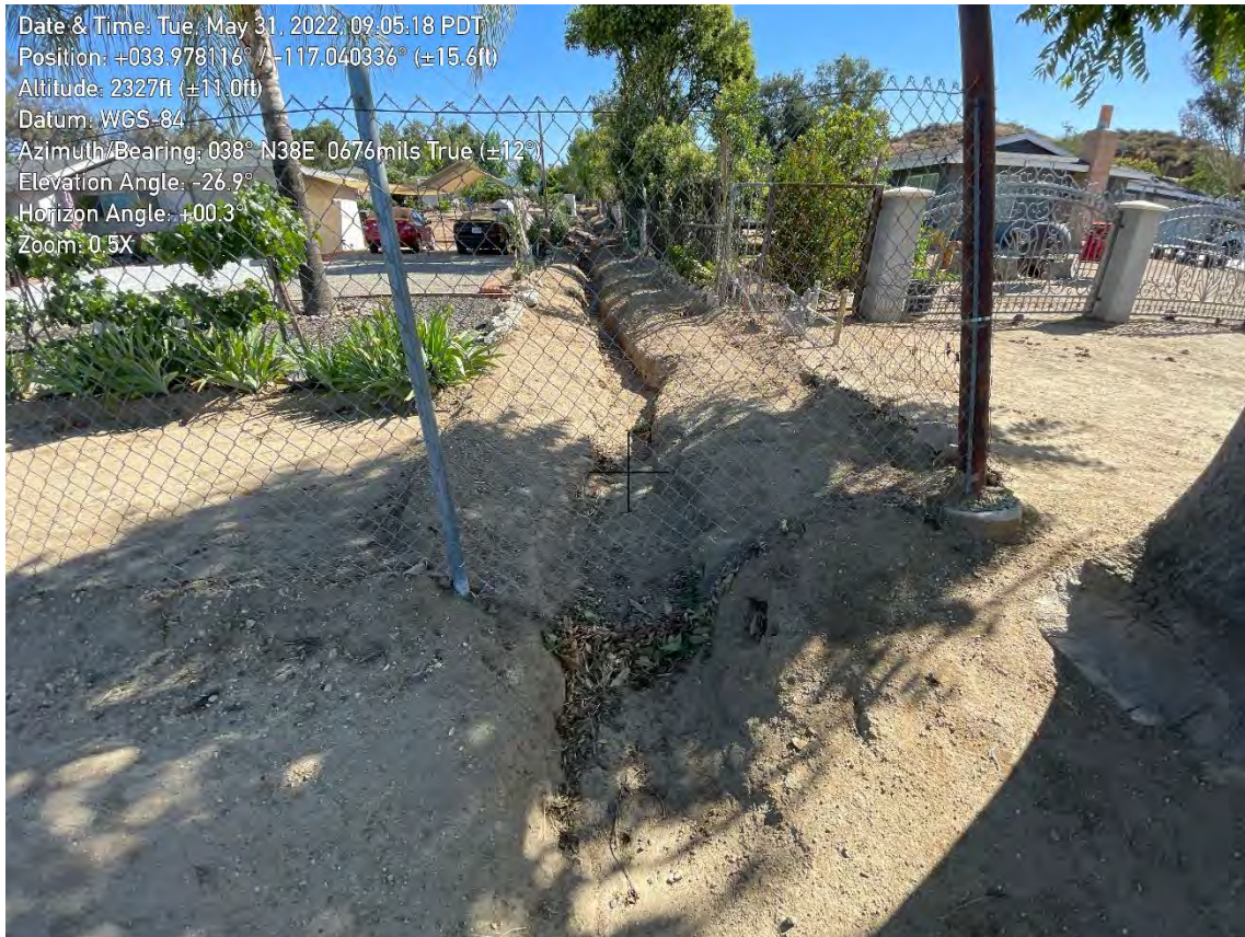
Upstream offsite excavated channel on residential property leading to D2 above the northern site boundary.
