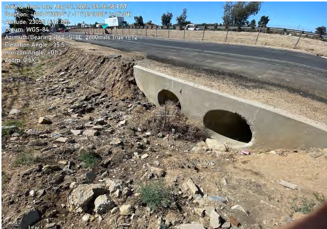
Inlet Structure (D3) facing southeast leading to under road crossing.
