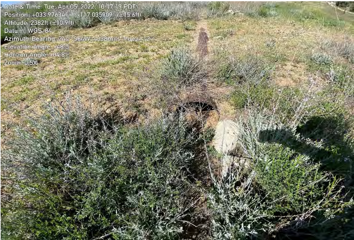
Portion of underground pipe, D4 facing southwest.
