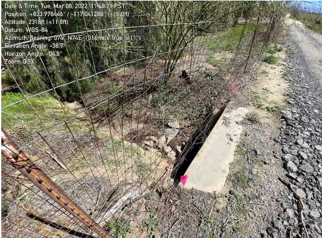
Upstream (offsite) view of D1 entrance to under road crossing and adjacent residential property.
