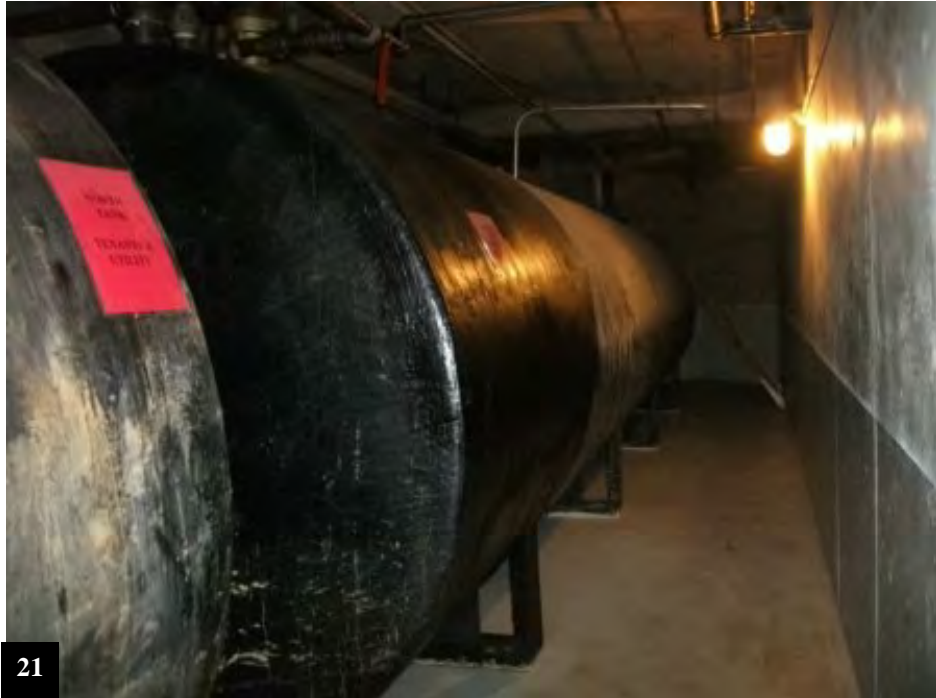
8,800-gallon diesel ASTs in secondary containment room
