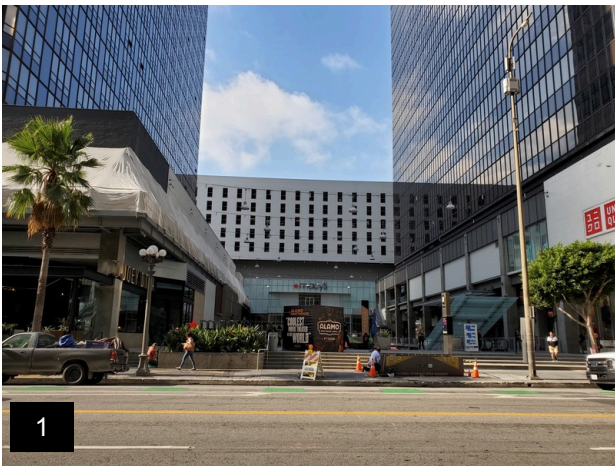
1 Northeast side of Subject Property
