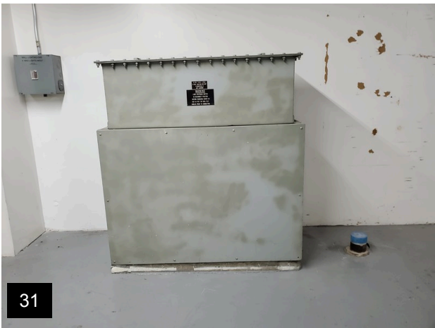
High voltage switch equipment - possible PCBs
