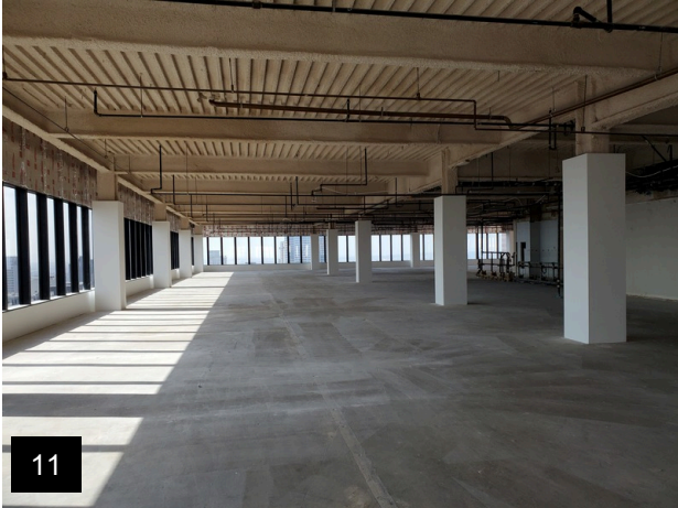
11 Floor 33 of office tower
