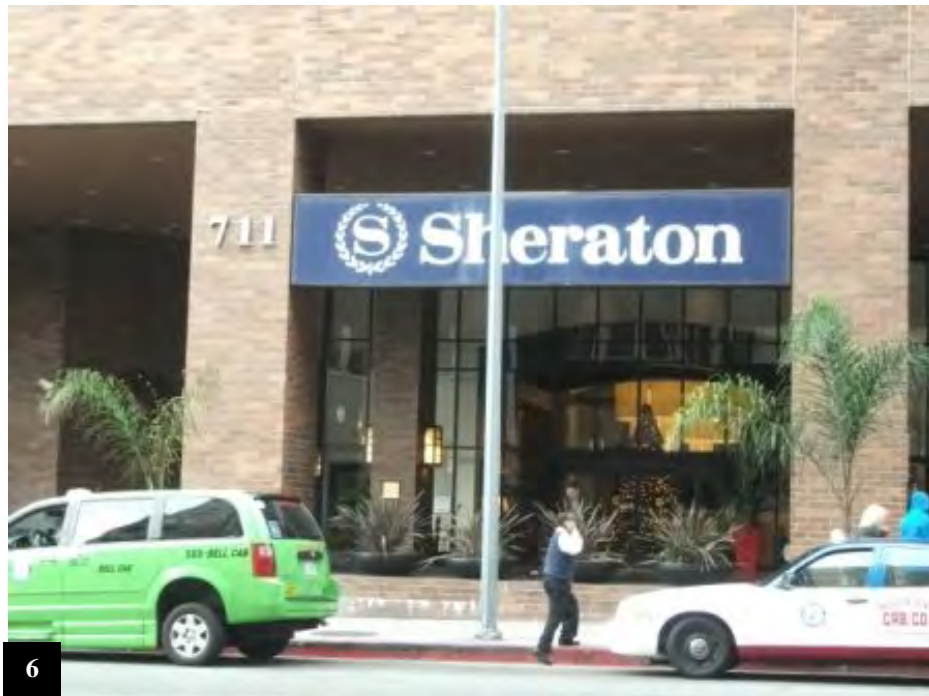
Entrance to Sheraton Hotel on S. Hope Street
