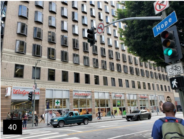
40 Adjacent property to east-northeast
