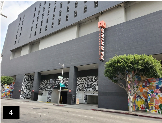
4 Southwest side of Subject Property
