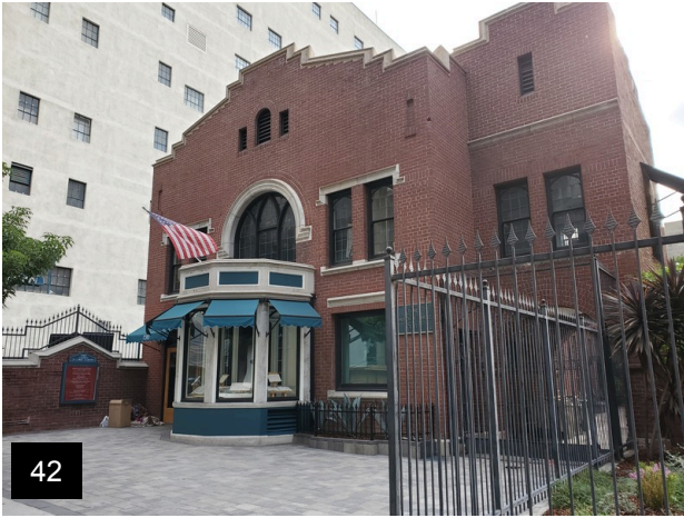
42 Adjacent property to southeast
