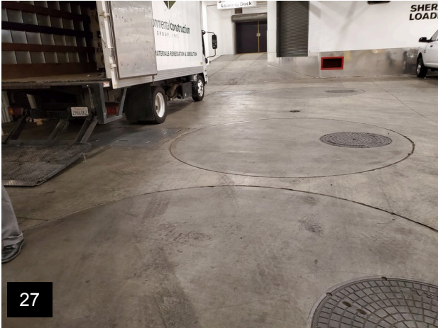
New stormwater sumps at loading dock
