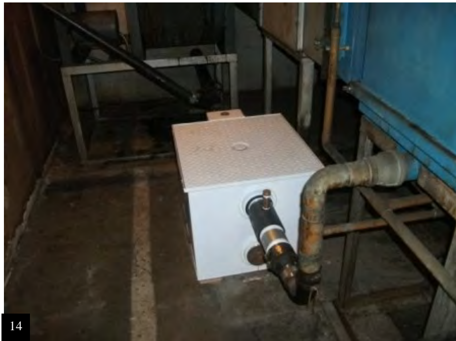
Typical grease trap
