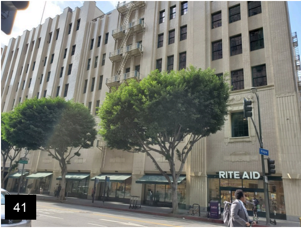
41 Adjacent property to southeast
