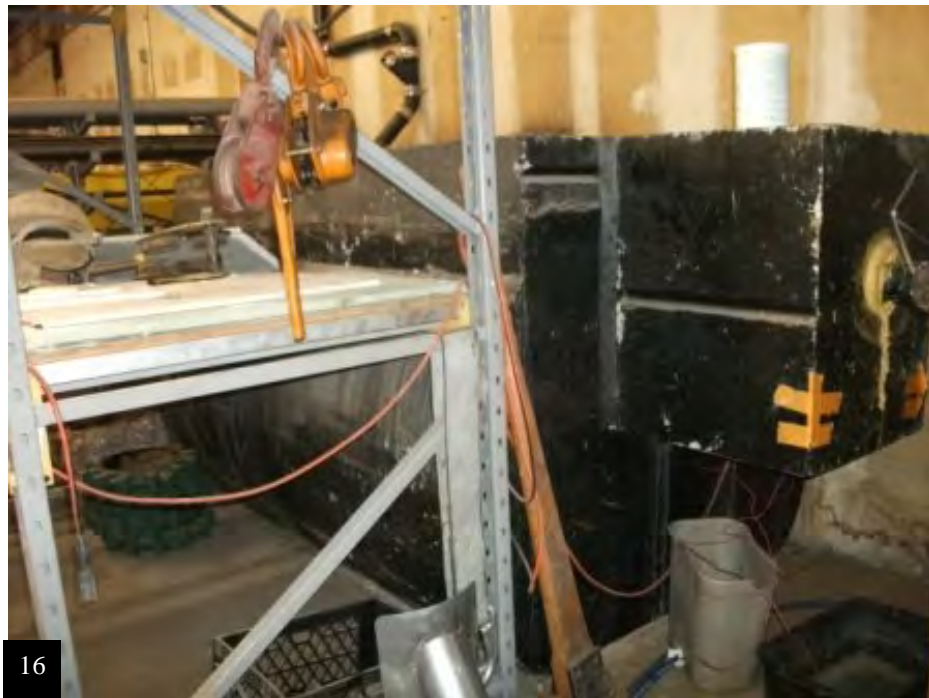
Car wash clarifier □ floor below car wash
