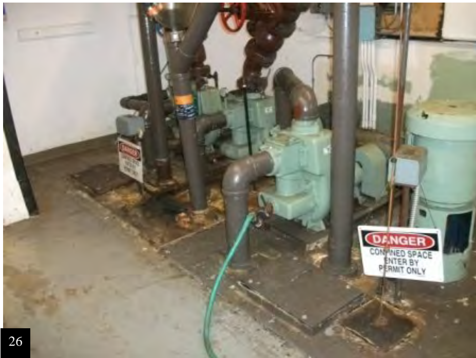
Storm water and sanitary sewer sumps
