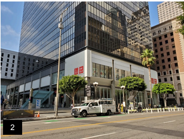
2 Northeast side of Subject Property office tower
