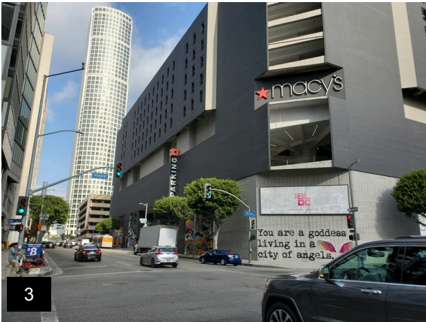
3 Southwest side of Subject Property
