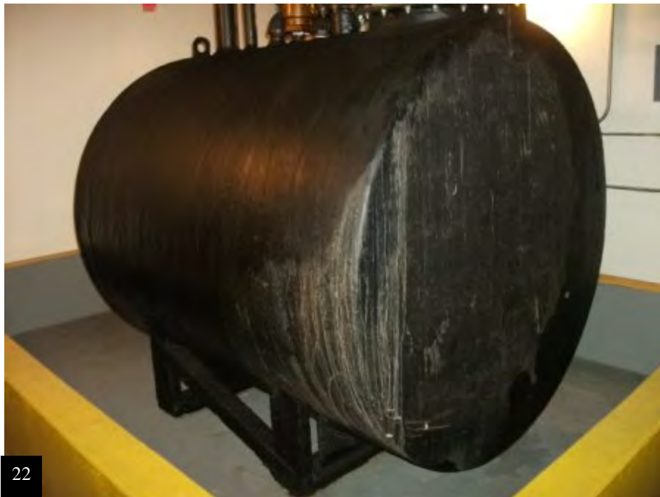
1,000-gallon diesel transfer AST
