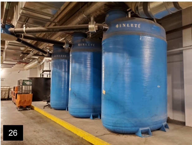
Grease interceptors at loading dock
