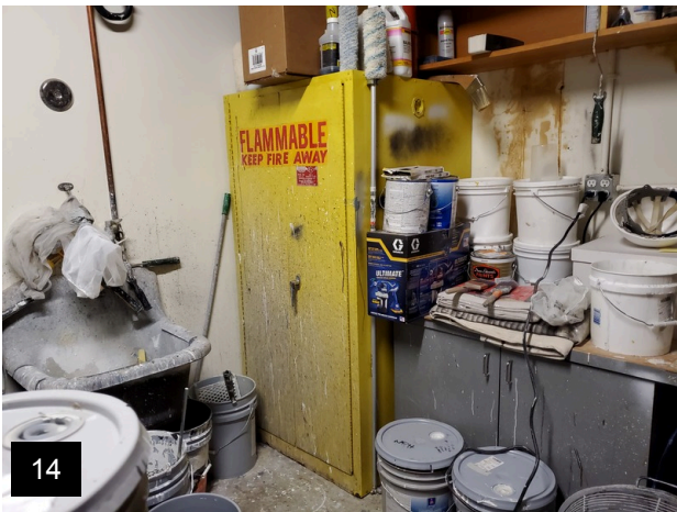
14 Chemical storage cabinet in maintenance area
