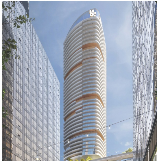
New Tower Top Sign - Facing Flower St / West Facade BDE-13 25'-8" w x 21'-3" h
