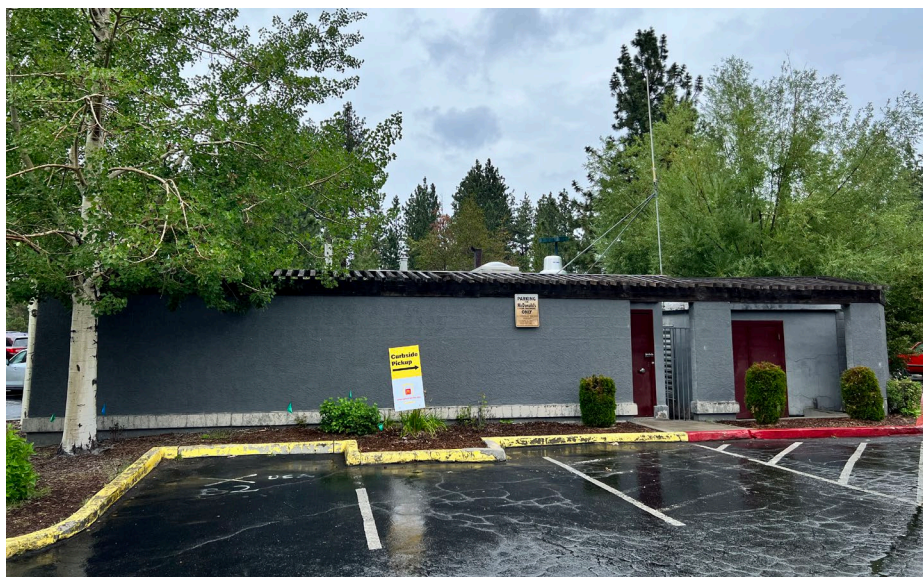
Figure 1 Existing Station. View is to the north.
