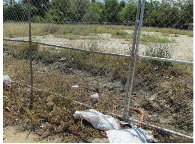
8. View of the stormwater drainage centrally located near the eastern boundary
