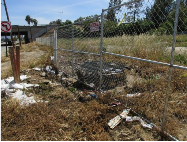
7. View of the stormwater drain centrally located near the eastern boundary
