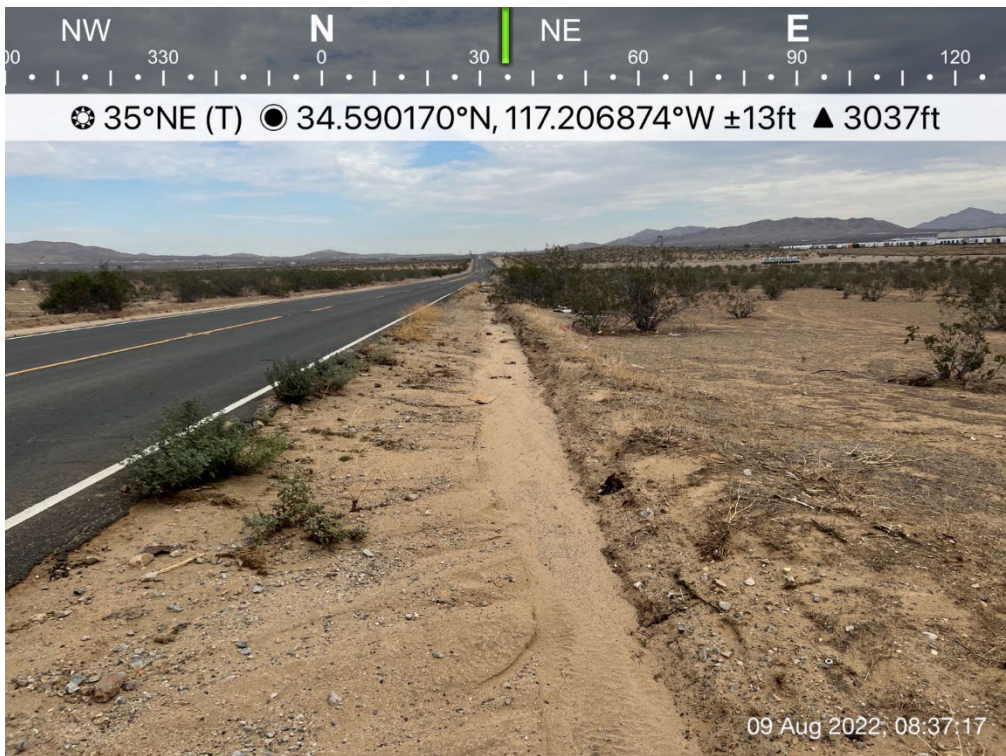
Photo 8. Looking north showing the roadside ditch along Dale Evans Parkway.
