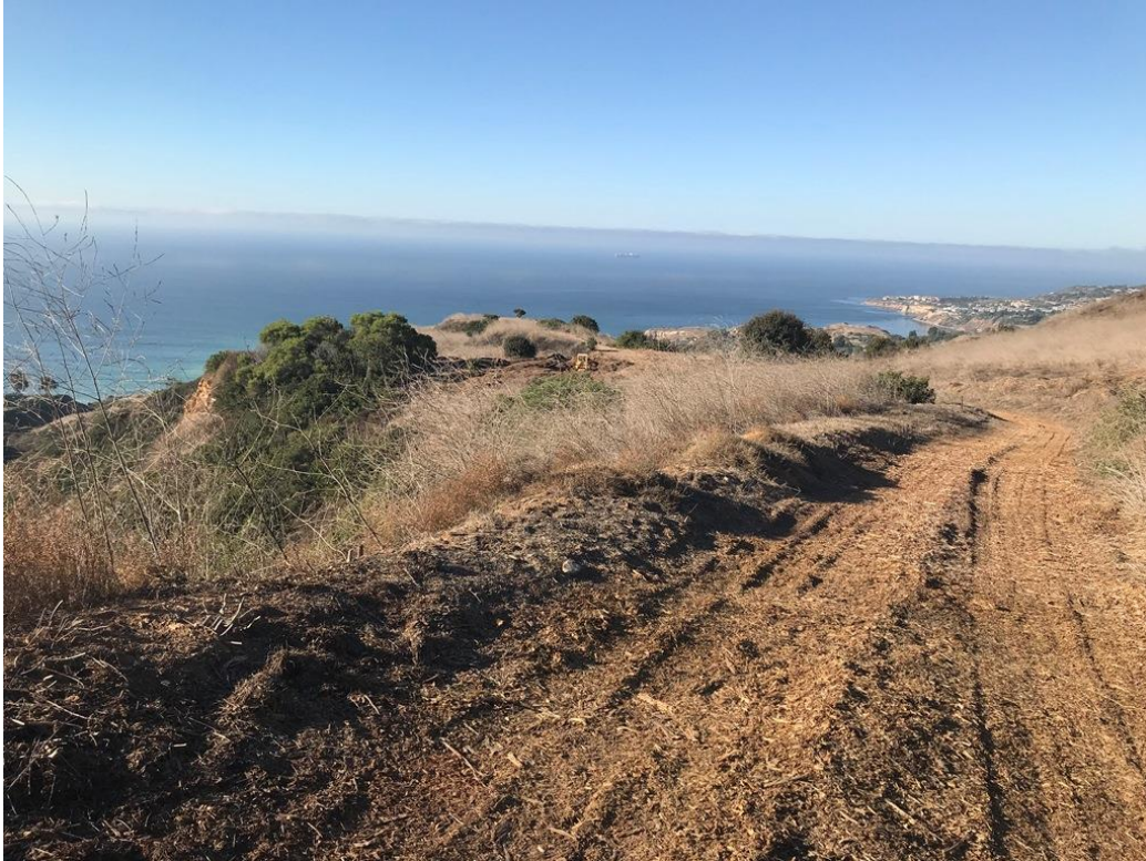
Photograph 1. View of the existing access road (Portuguese Bend Road), facing west
