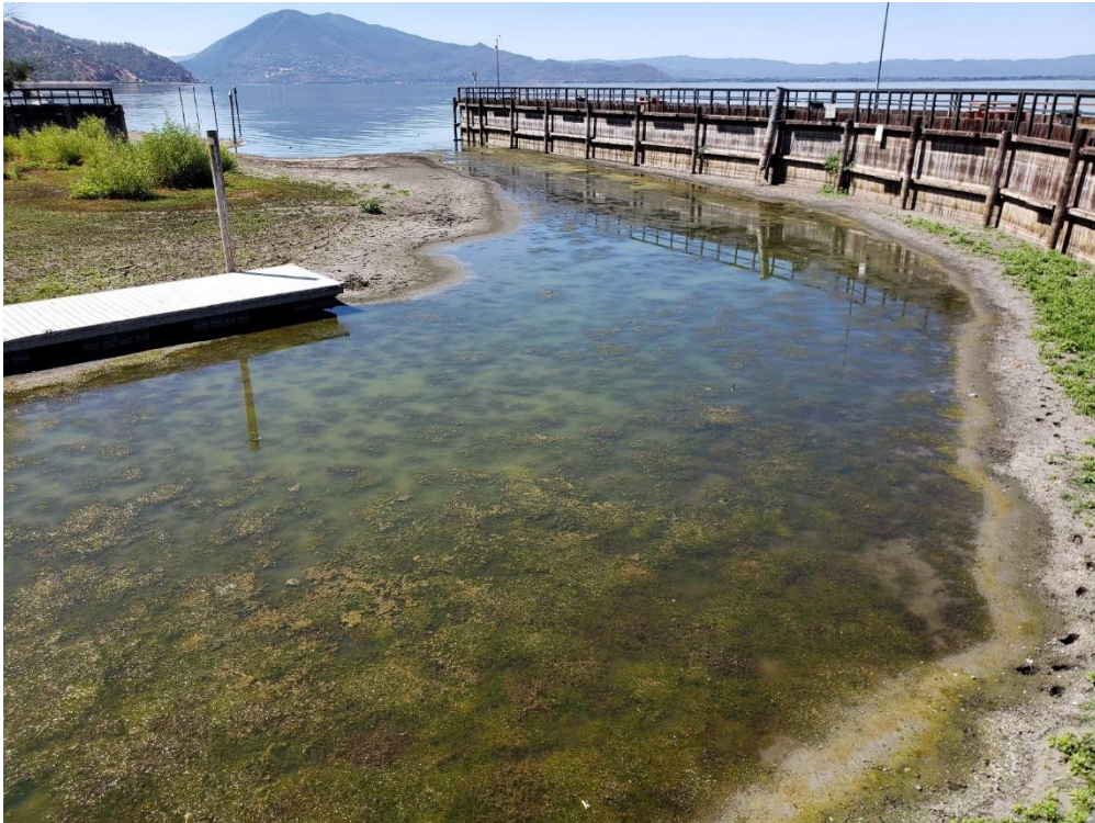
Photo 2: View of harbor entrance
