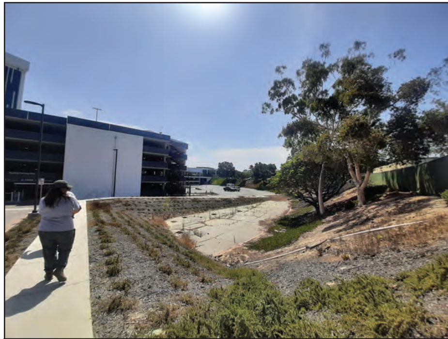
① View from the north side of the project site on Del Amo Circle Way looking southeast towards the rest of the project site.
