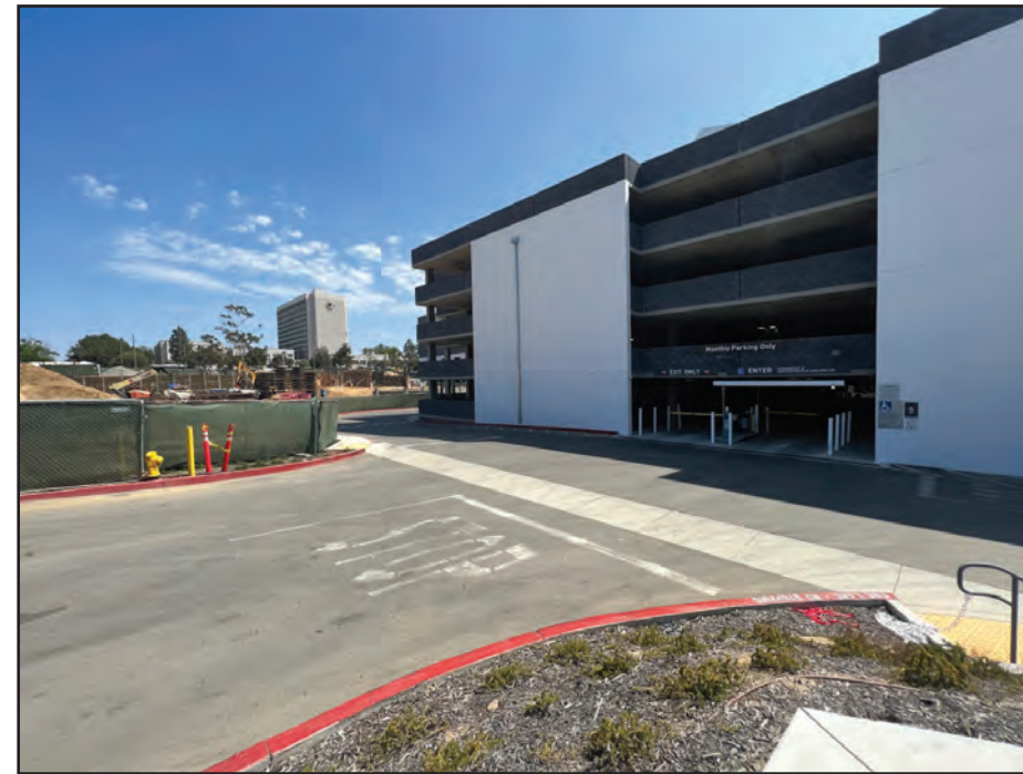
2 View from northwest corner of the project site looking northeast towards the west side of the Del Amo Crossing parking structure.
