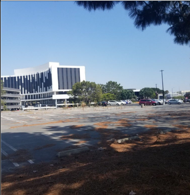
Photograph 3: View of the Site looking east from the SW corner.
