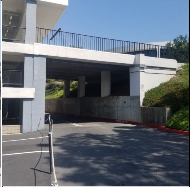
Photograph 18: View looking east from the northeast corner of the Site.
