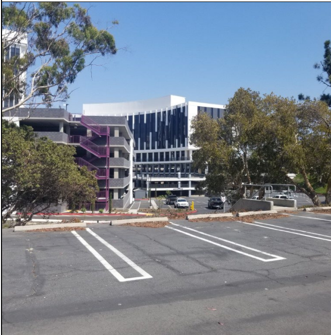
Photograph 15: View east from the northwest portion of the Site.
