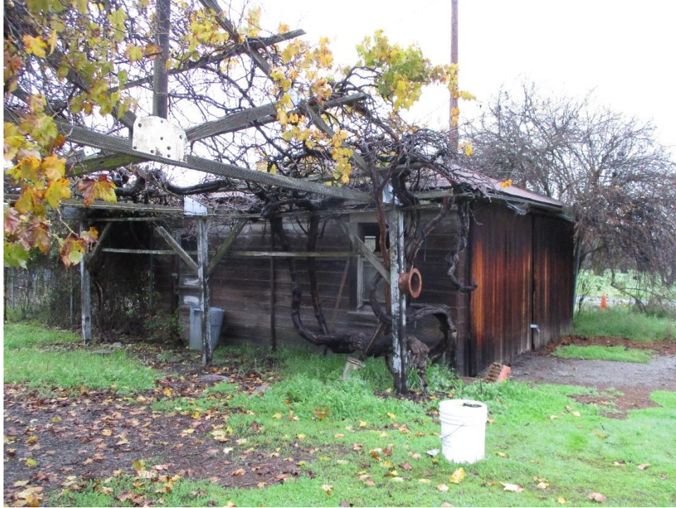
Figure 48. West and south elevations of the ca. 1923 garage, facing northeast.
