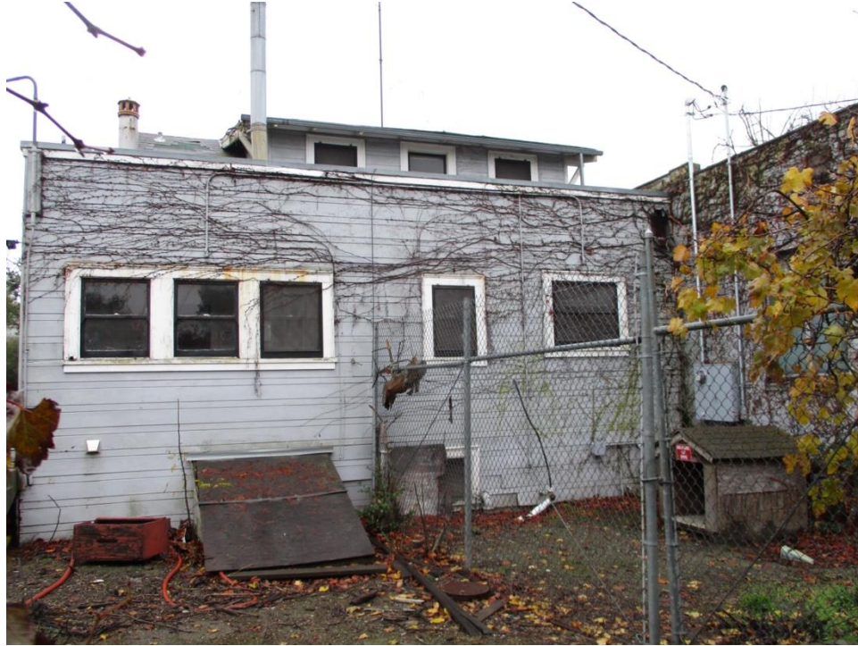
Figure 39. East wall of north elevation.
