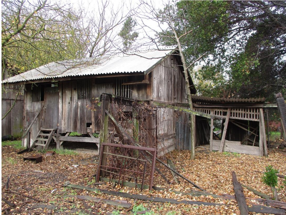
Figure 71. South and east elevations of the ca. 1923 chicken coop, facing northwest.
