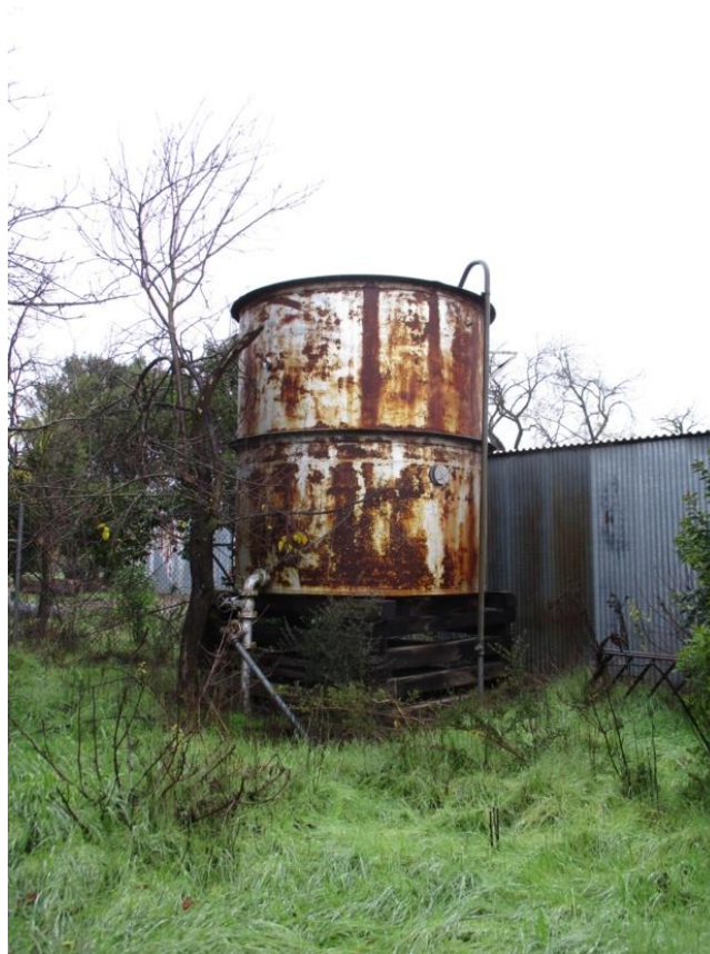
Figure 46. Tank house 2, facing northeast.
