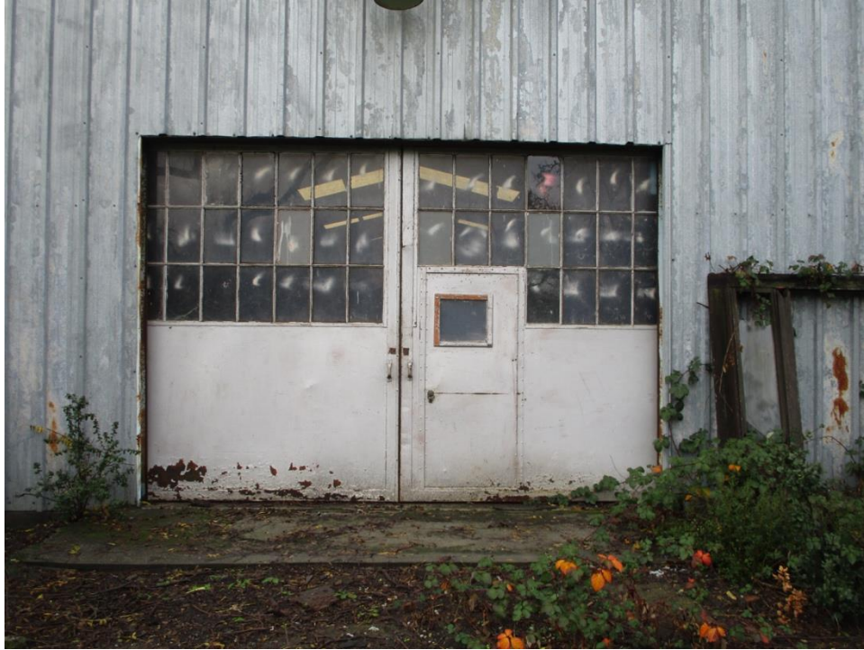
Figure 62. West elevation of the ca. 1970 barn, facing east.
