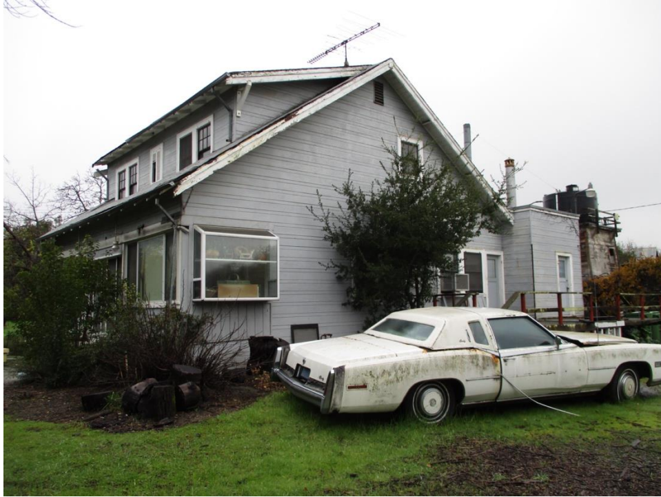
Figure 34. East elevation, facing northwest.
