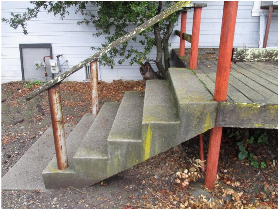
Figure 37. Concrete stairs to patio on east elevation, facing west.
