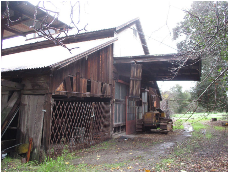
Figure 1. West elevation of the ca. 1923 walnut barn, facing southeast.
