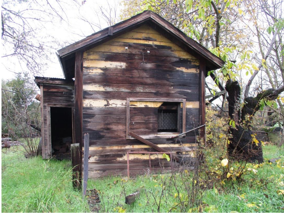
Figure 66. South elevation of the 1927 San Ramon rail depot, facing east.
