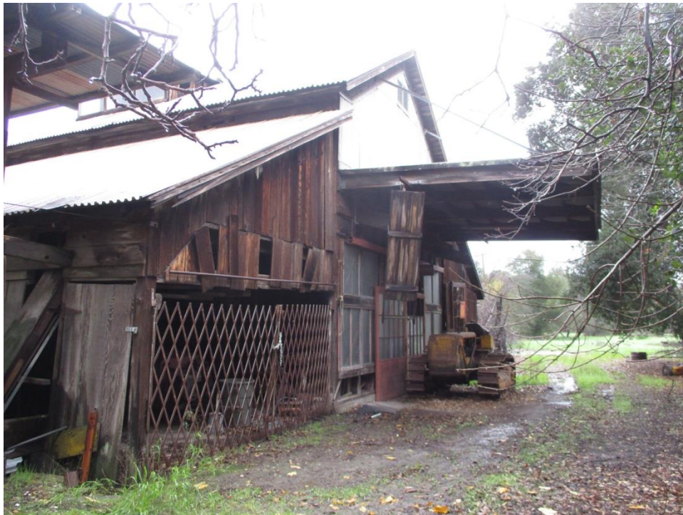
Figure 52. West elevation of the ca. 1923 walnut barn, facing southeast.
