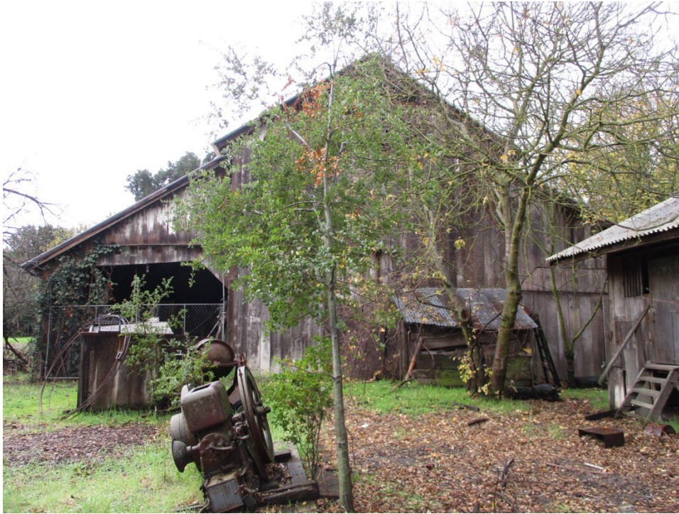
Figure 4. East elevation of the ca. 1923 walnut barn, facing west.
