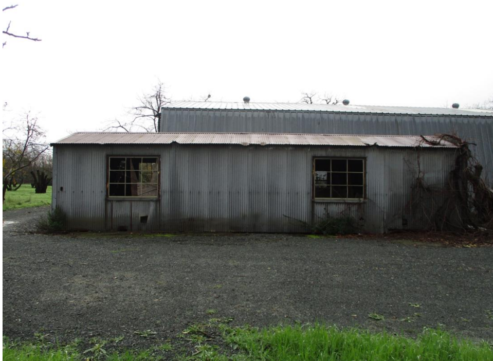
Figure 70. North elevation of the ca. 1960 gable building, facing south.
