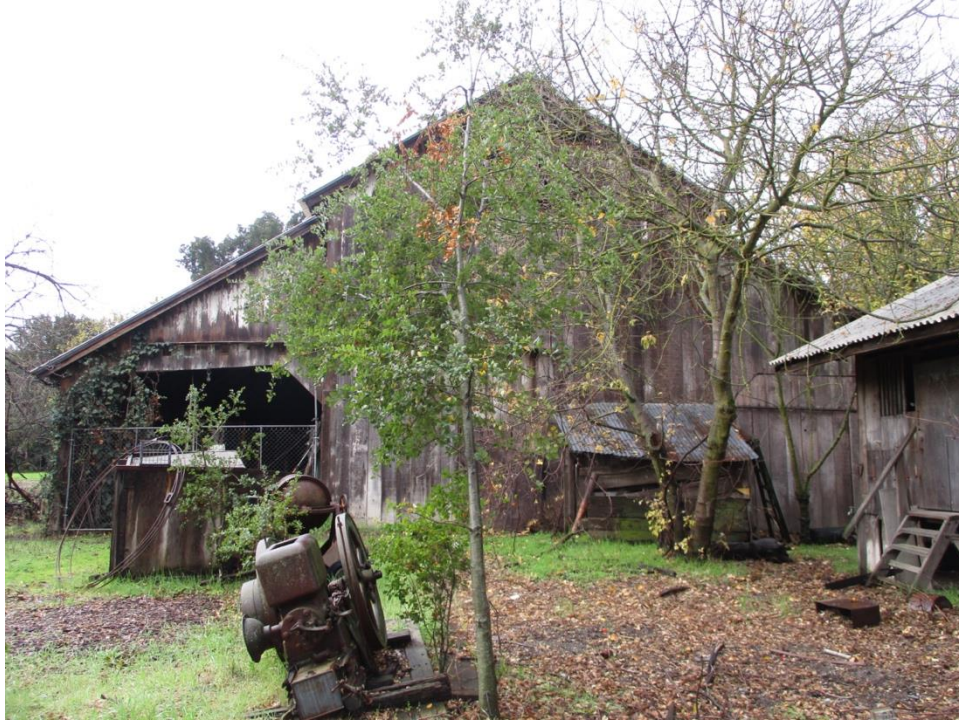
Figure 55. East elevation of the ca. 1923 walnut barn, facing west.
