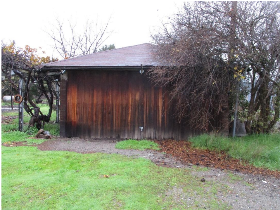
Figure 49. South elevation of the ca. 1923 garage, facing north.
