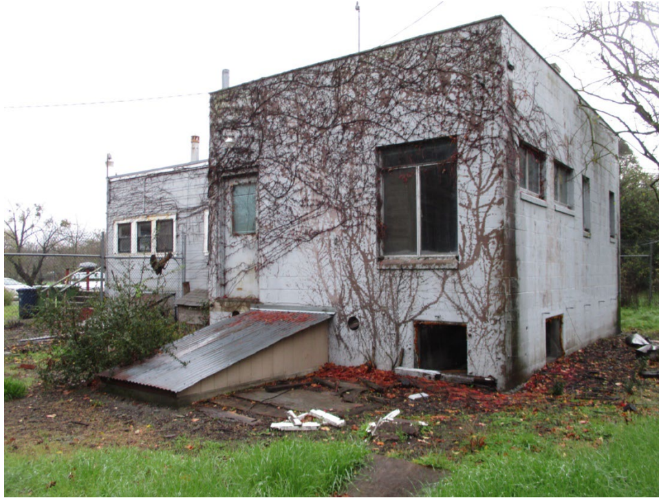
Figure 9. North elevation, facing southwest.
