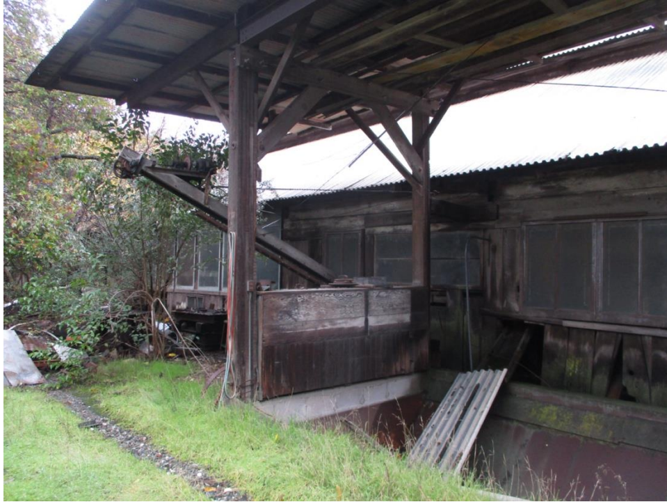
Figure 57. Close-up view of the timber elements of the awning.
