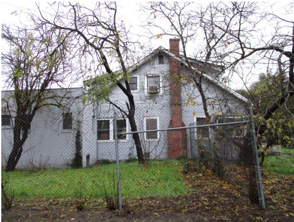
Figure 10. West elevation, facing east.
