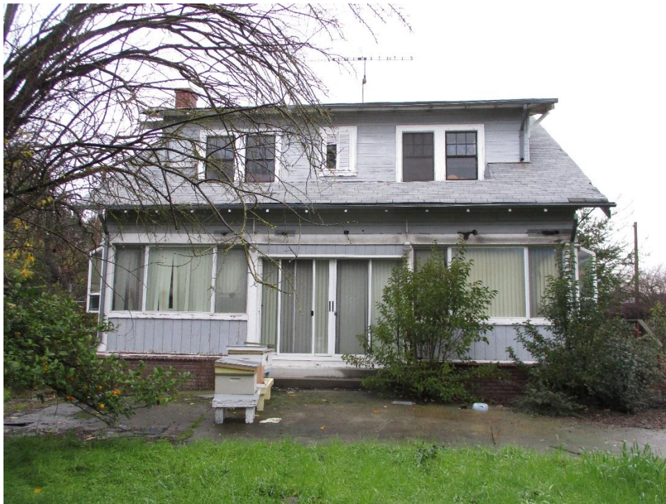
Figure 32. South elevation, facing north.
