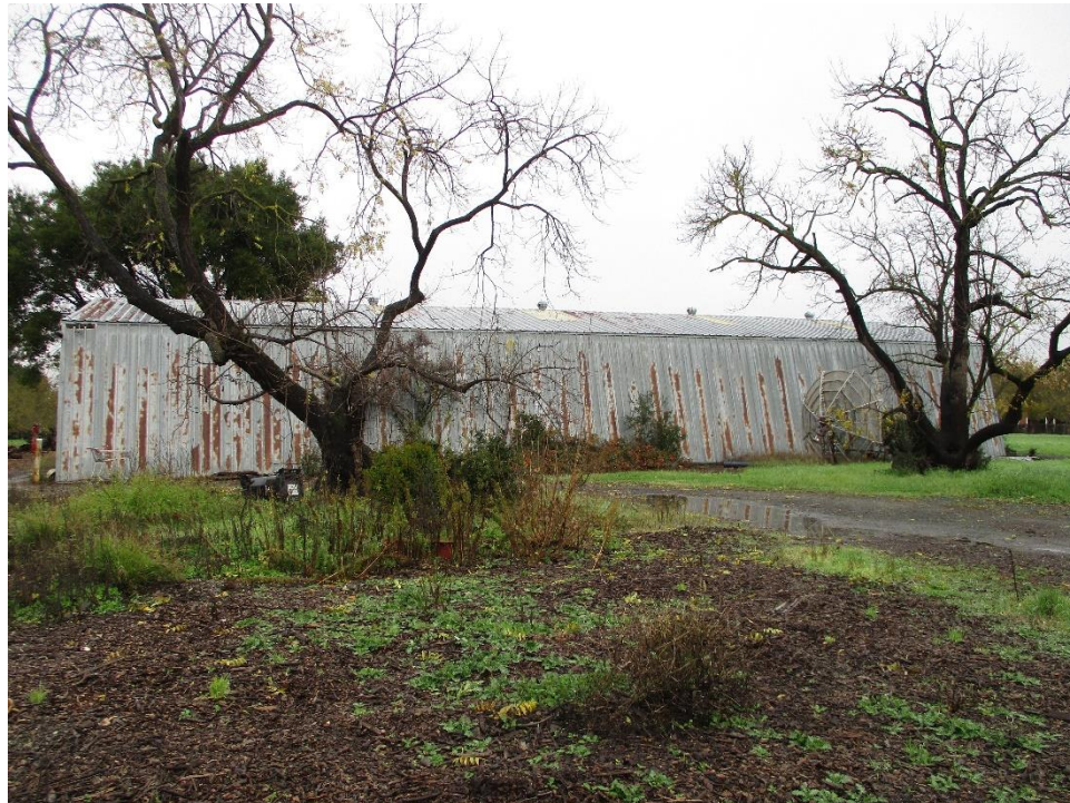
Figure 63. South elevation of the ca. 1970 barn, facing north.
