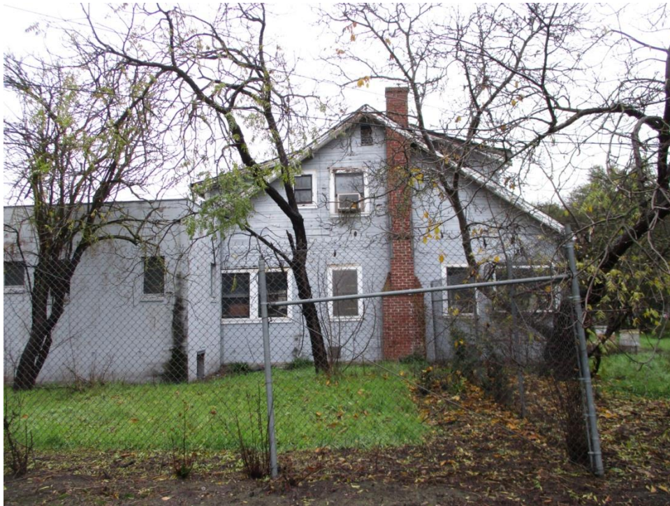
Figure 41. West elevation, facing east.
