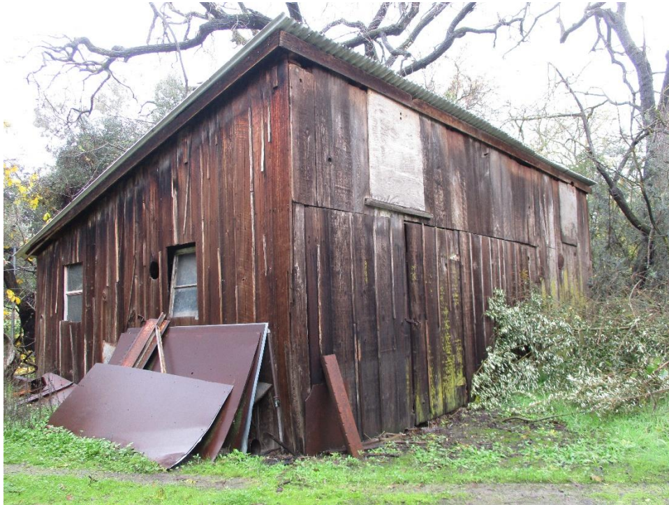
Figure 65. South and east elevations of ca. 1923 shed building, facing northwest.
