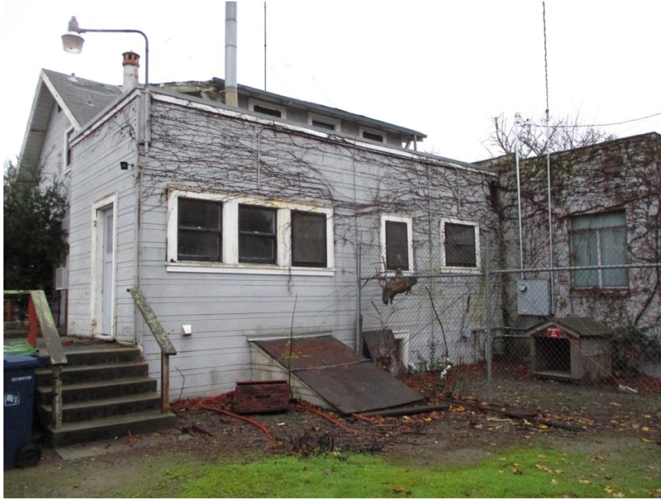
Figure 36. North and west elevations of two additions, with storm cellar entry.
