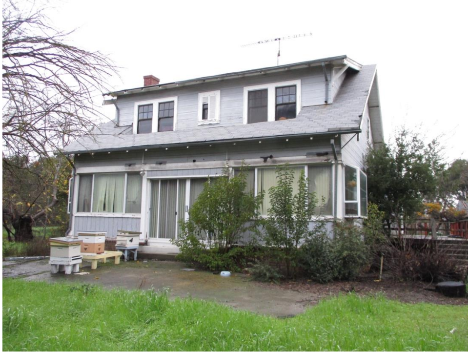
Figure 31. Southeast corner of house, facing northwest, demonstrating the first phase of construction.
