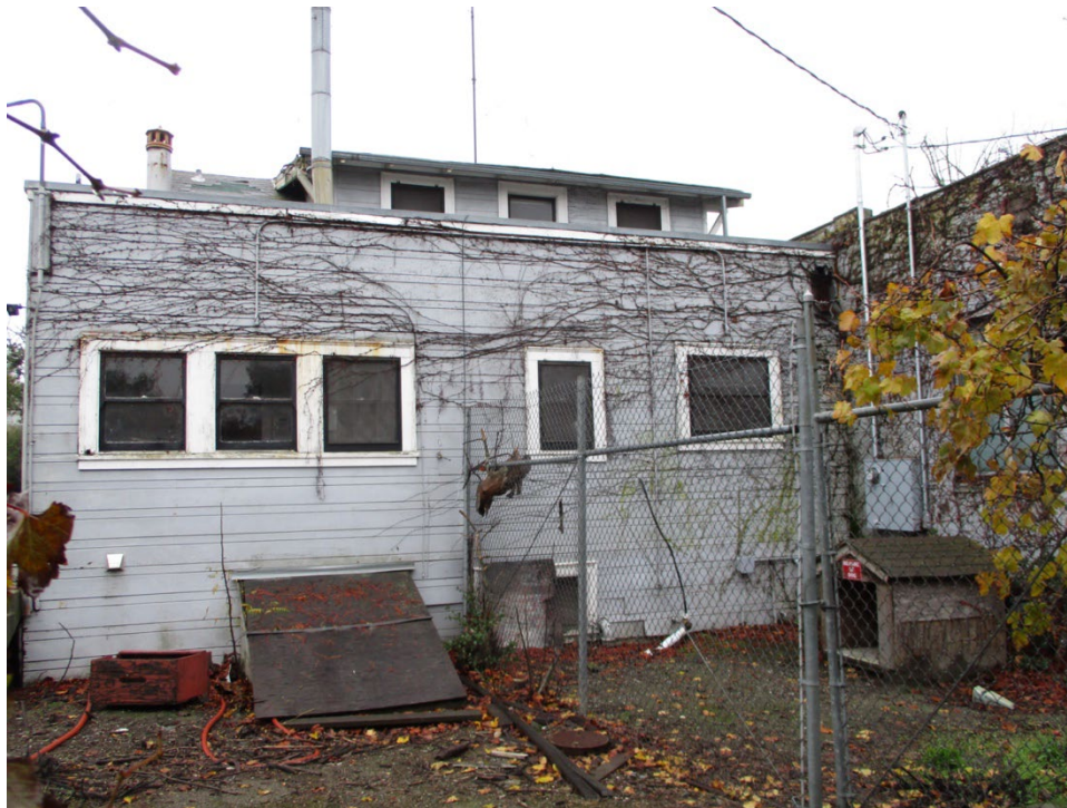
Figure 8. East wall of north elevation.
