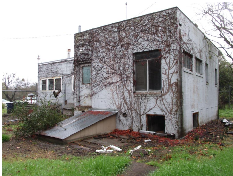
Figure 40. North elevation, facing southwest.
