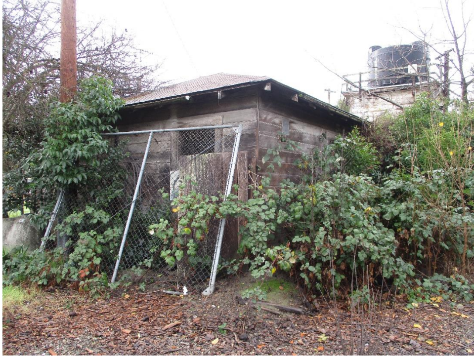
Figure 50. North and east elevations of the ca. 1923 garage, facing southwest.
