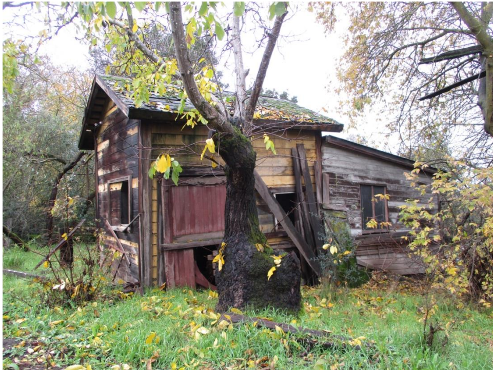
Figure 67. East and south elevations of the 1927 San Ramon rail depot, facing west.
