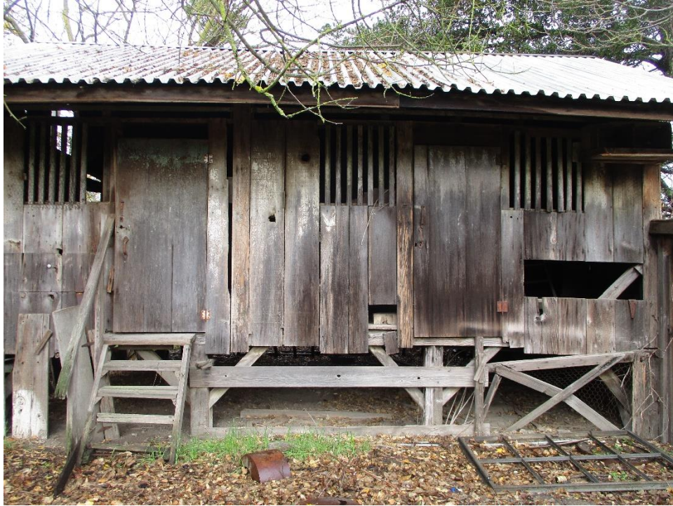
Figure 72. South elevation of the ca. 1923 chicken coop, facing north.
