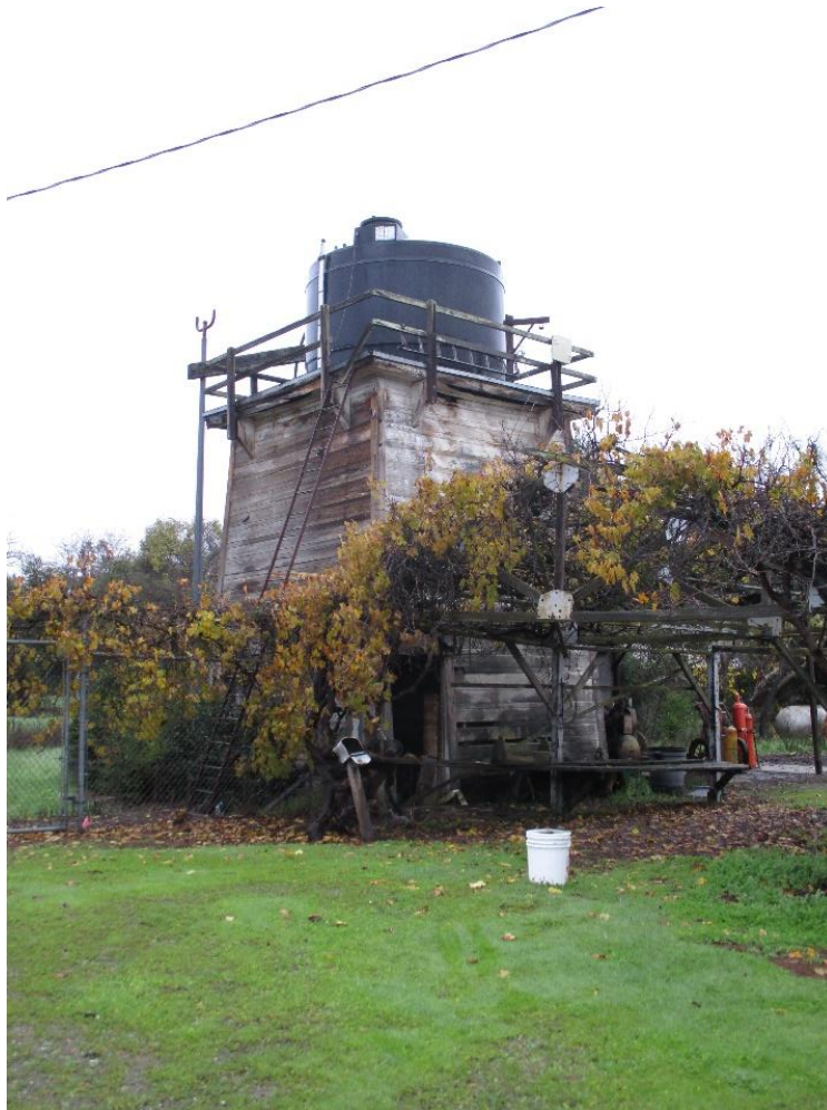
Figure 44. Tank house 1, facing northeast.
