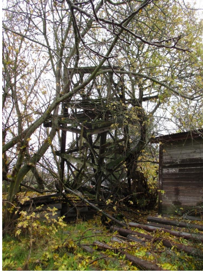
Figure 47. Remnants of tank house 3.
