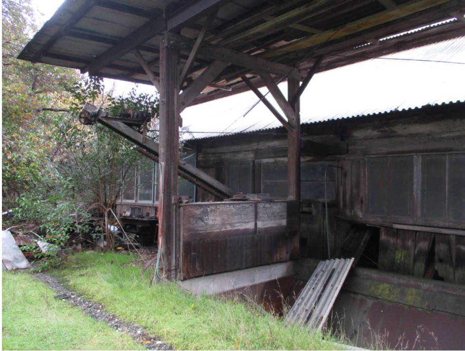
Figure 6. Close-up view of the timber elements of the awning.
