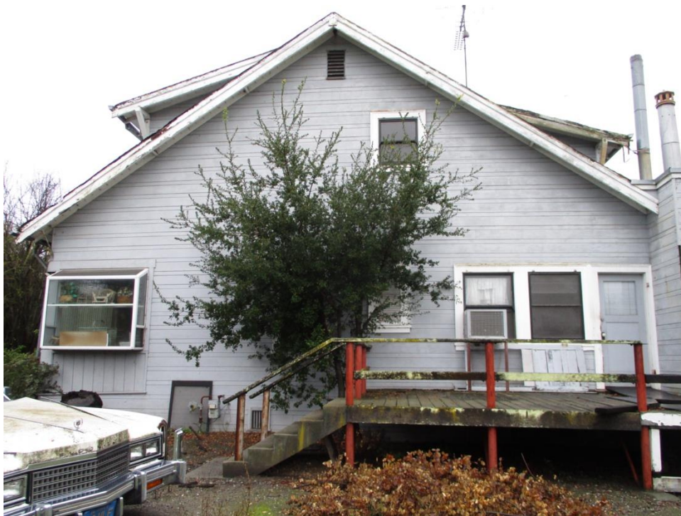
Figure 35. East elevation showing the raised patio deck, facing west.
