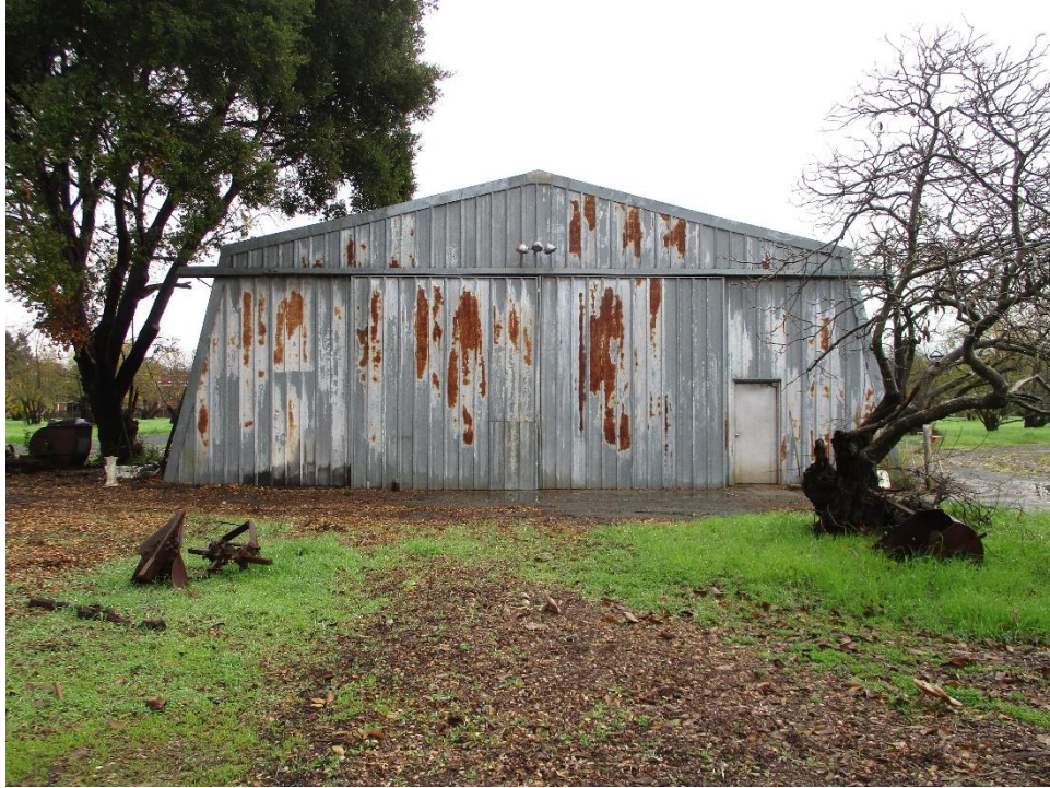
Figure 64. East elevation of the ca. 1970 barn, facing west.
