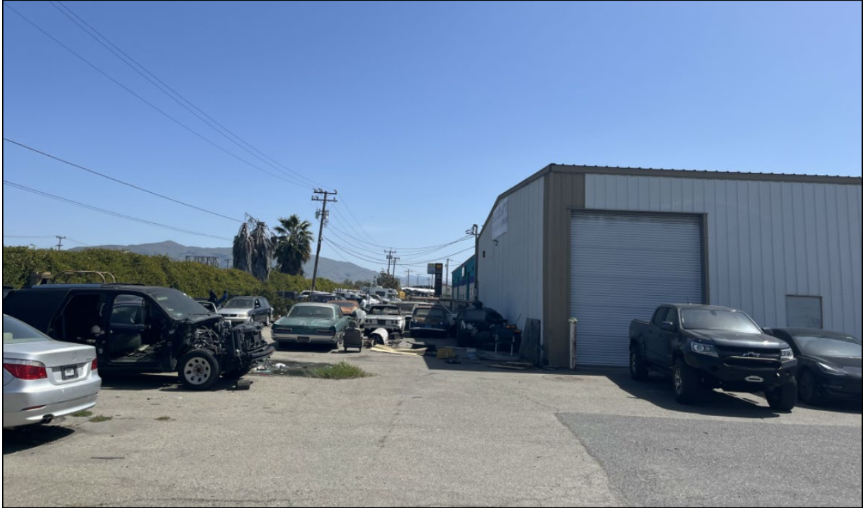
Figure 3.d- Looking south at the rear of the project site behind the building at 38486 Cedar Blvd within the site.
