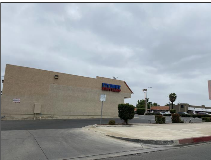
17. View of the east adjoining property
