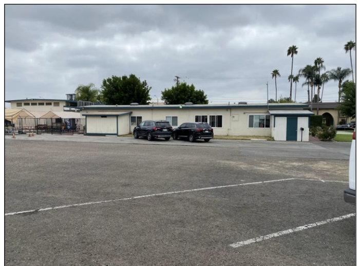
12. View from the northwest corner facing south
