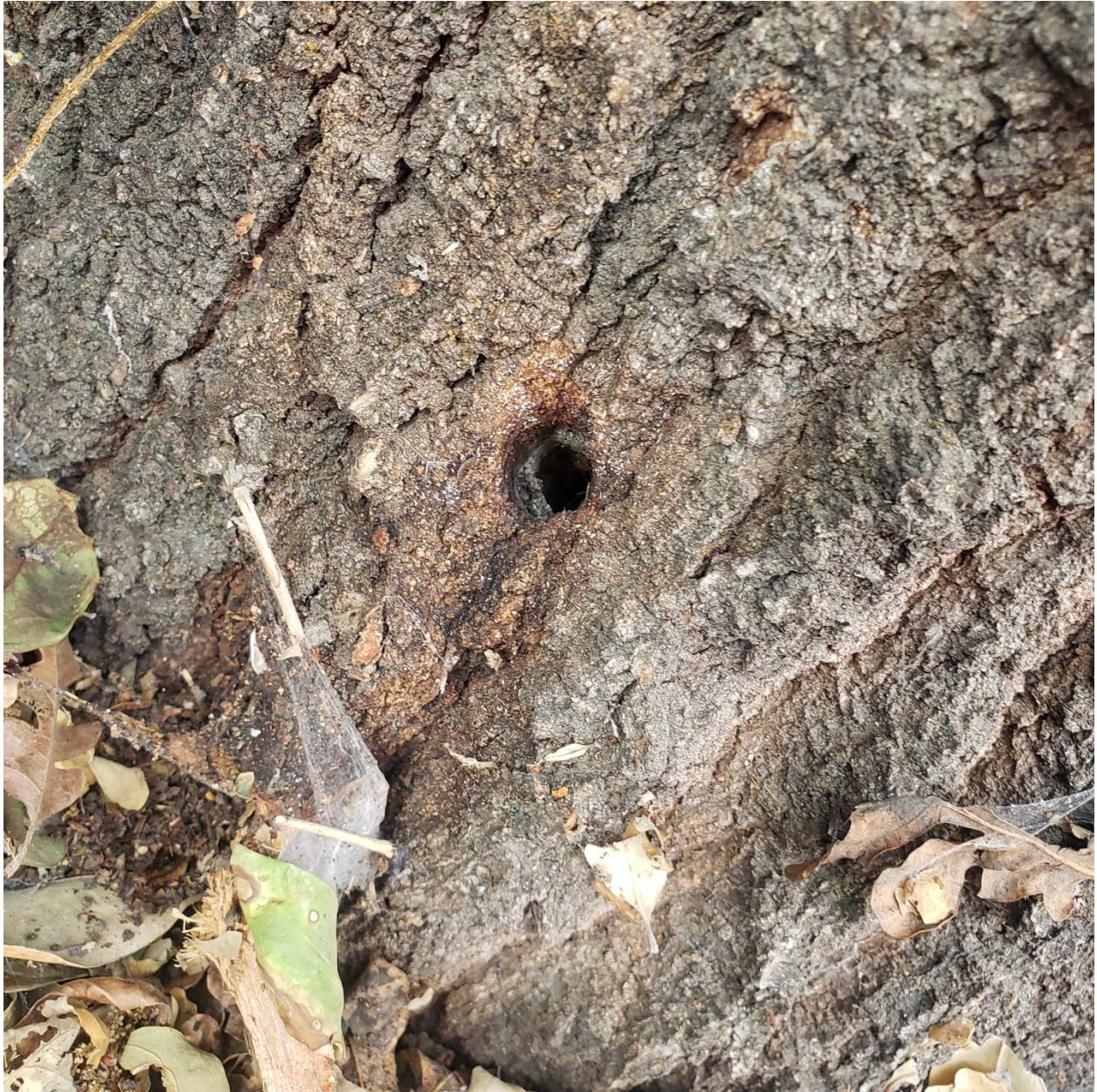
Photo 3: Hole drilled into the east side of the base of the tree (# 297). The hole is approximately \frac{3}{4} " in diameter.
