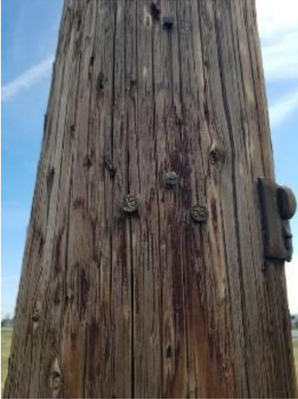
**Photo 3:** close up of utility pole inspection tags; UTM 11S 458051mE 3777254mN
