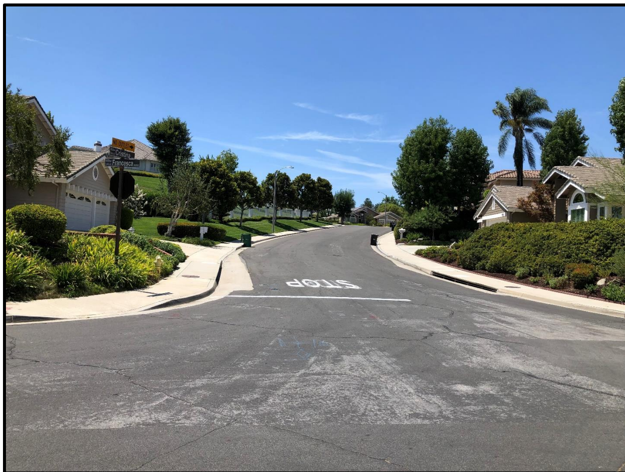
Figure 4.3-2 CALLE CRISTINA AT CALLE FRANCESCA; VIEW TO THE WEST
