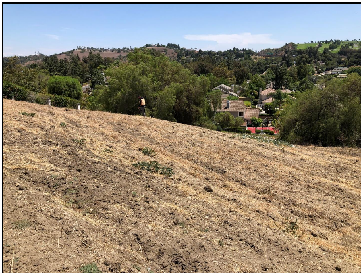
Figure 4.3-4 SURVEYED SLOPE ON SOUTH SIDE OF CALLE CRISTINA; VIEW TO THE SOUTHEAST
