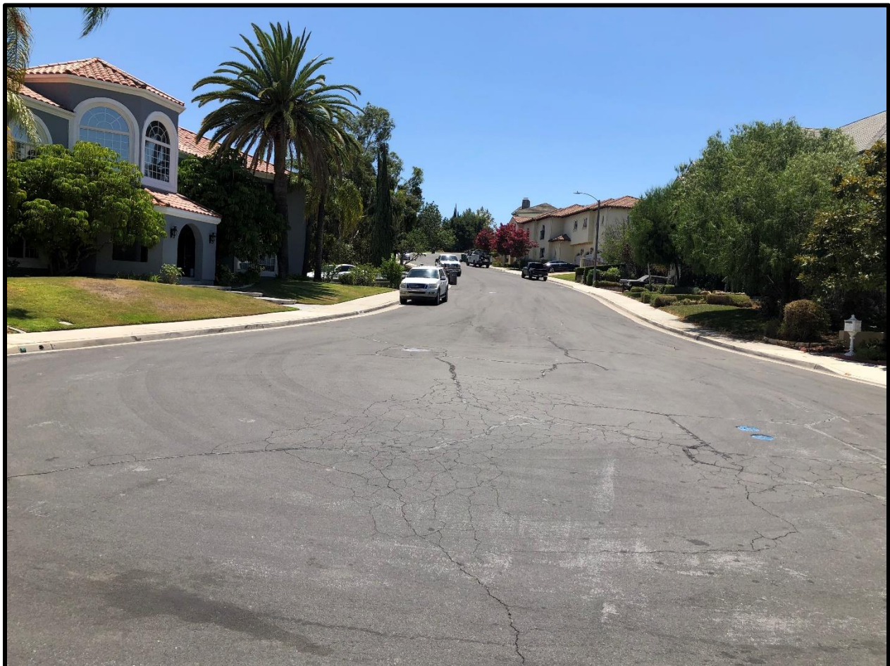
Figure 4.3-1 CALLE CRISTINA FROM NOTH END; VIEW TO THE SOUTHWEST
