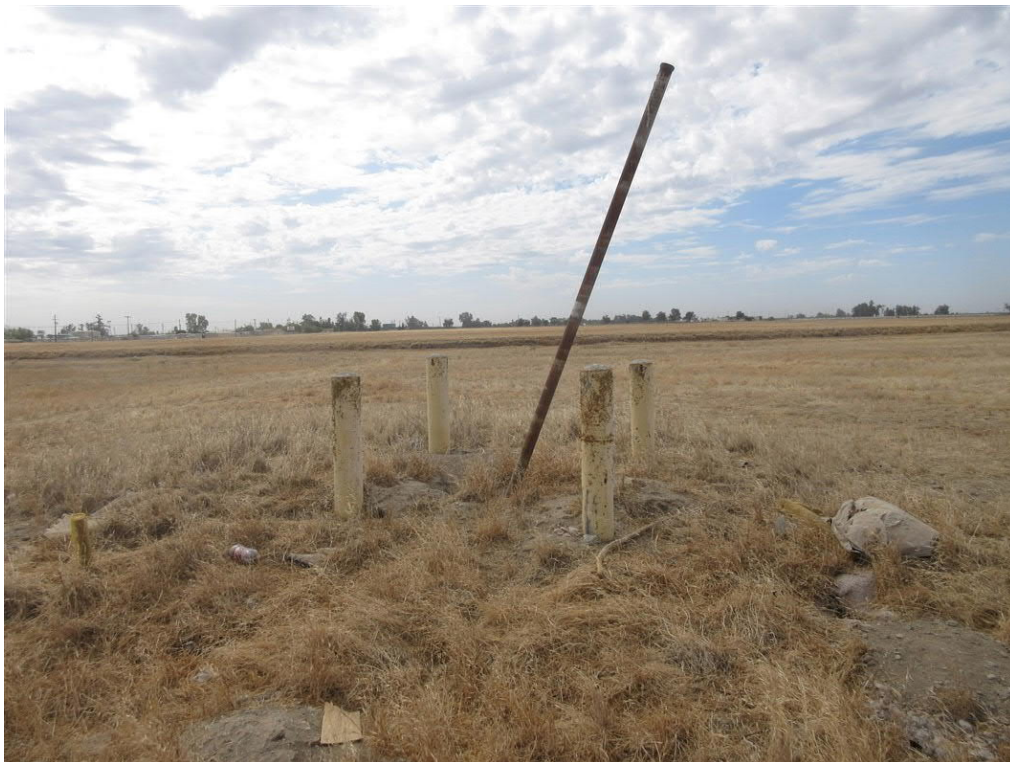
Photo 12: View of a capped steel pipe protruding from the ground surface located in the central portion of the subject site.
