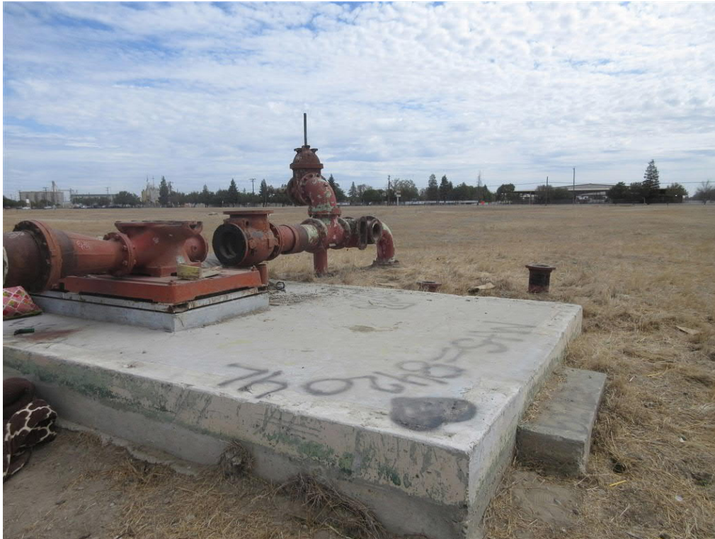
Photo 11: View of the water conveyance feature and potential water well located in the central portion of the subject site.
