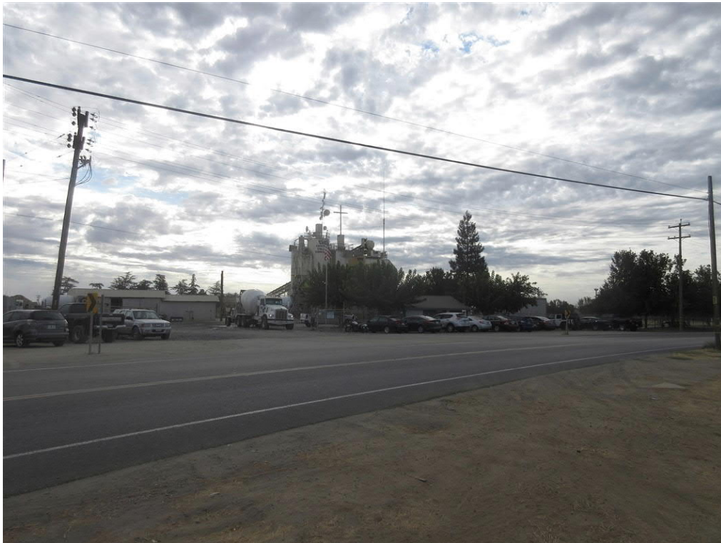
Photo 14: View of the concrete batch plant located adjacent to the east of the northern portion of the subject site.
