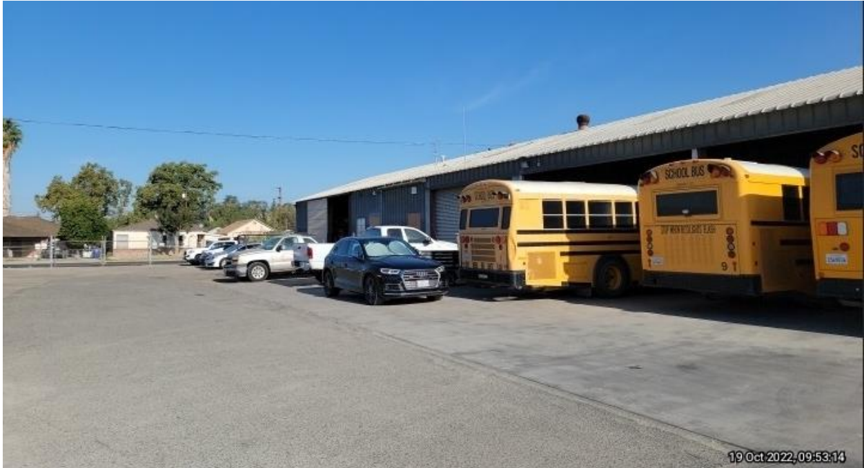
Figure 10 Subject Building; Maintenance, Operations and Transportation Building, Facing Northwest
