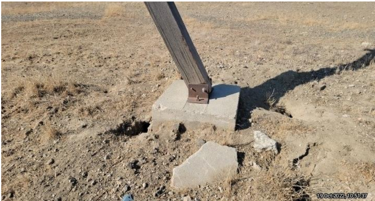
Figure 6 Concrete and Wooden Debris in Project Site, Proposed Athletic Fields, Facing West
