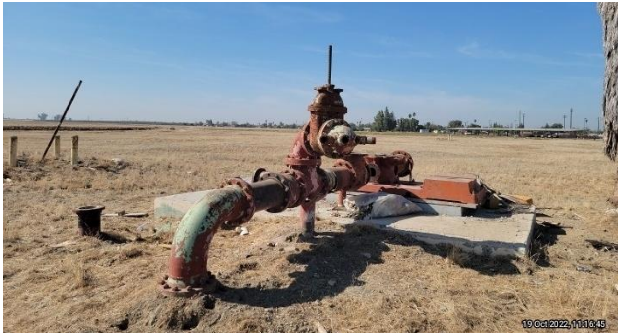
Figure 8 Pipe, Concrete Pad, and Metal Debris in Project Site, Proposed Athletic Fields, Facing Southwest
