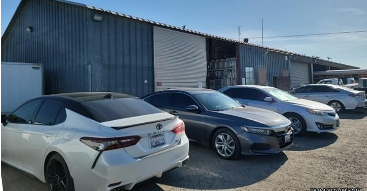
Figure 9 Subject Building; Maintenance, Operations and Transportation Building, Facing East
