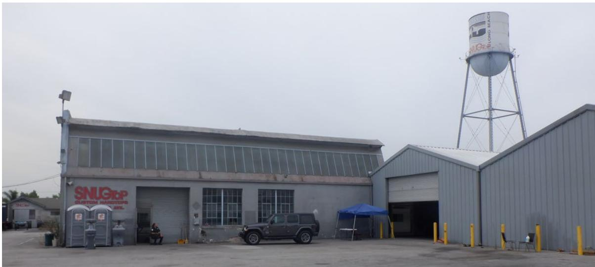
Photo 7. Eastern wing along Harbor Avenue with ribbon skylights and enframed metal sash windows (center). At right are two warehouses added to the northeast corner of the building complex in 2003. (Michael Baker International 9/9/2022)
