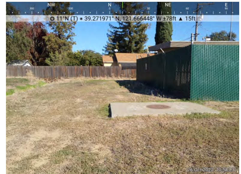
Photo 4. Disturbed Habitat with Existing Lift Station Facility
