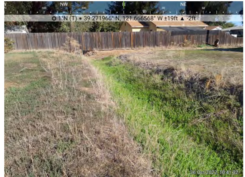
Photo 2. Constructed Stormwater Ditch
