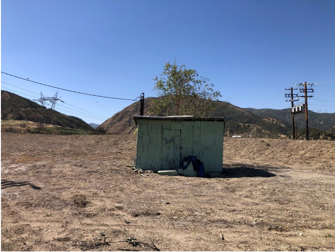
Figure 5-5. View of well shed, facing north.
