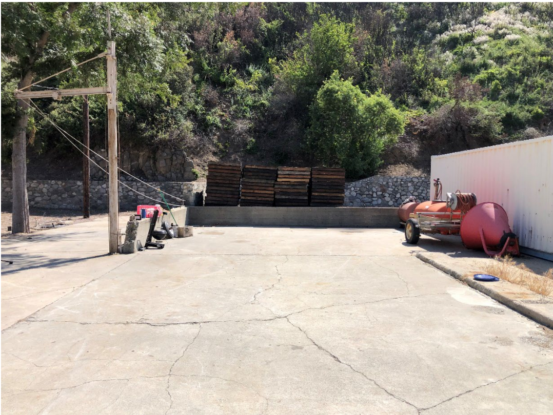
Figure 5-6. View of concrete slab with block and tackle, facing west.
