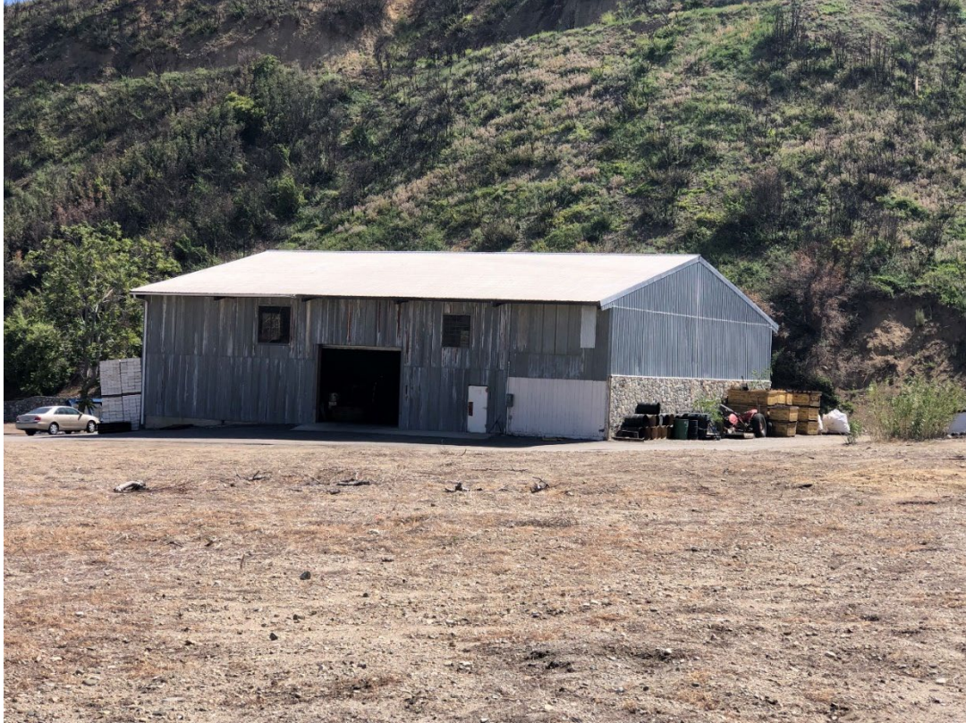
Figure 5-3. View of barn, facing southwest.
