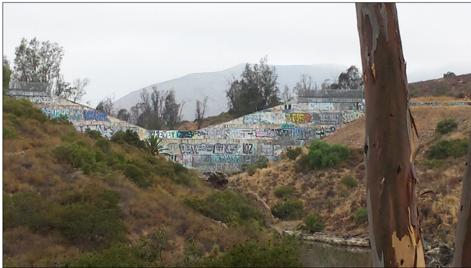
Plate 14. Overview of Upper Otay Dam and vicinity. View to the north.
