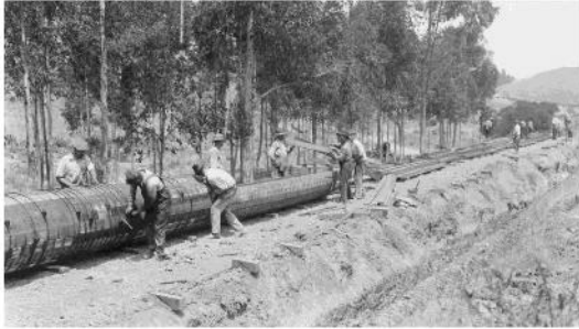
The construction of wood stave pipe near Chollas.
