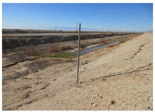
Plate 3. View northwest from Check 11 north from east side of Coachella Canal showing old canal with some remaining water in foreground and newer concrete-lined canal in background.
