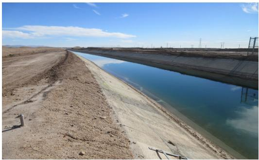
Plate 2. View south from center berm between original and lined canals; concrete-lined canal on right.
