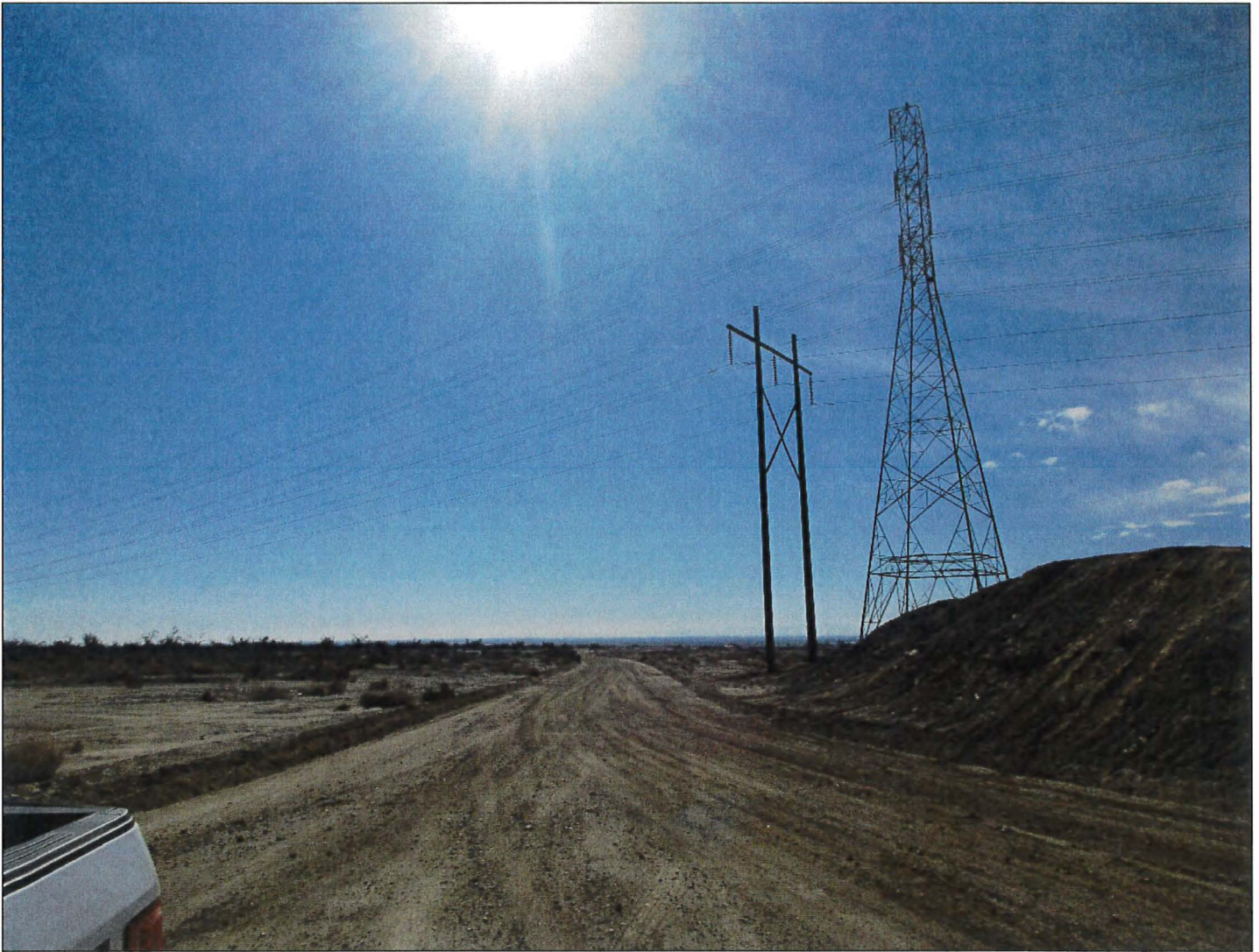
New single-phase primary line extension would need to cross under the IID's existing "KN&KS" 230kV and "N" 161kV transmission lines and proceed in a north westerly direction along the north side of the Coachella Canal Road right of way.
