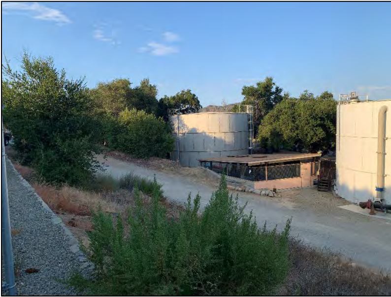
a. Baldwin tanks (north tank in photo center) and pump building
