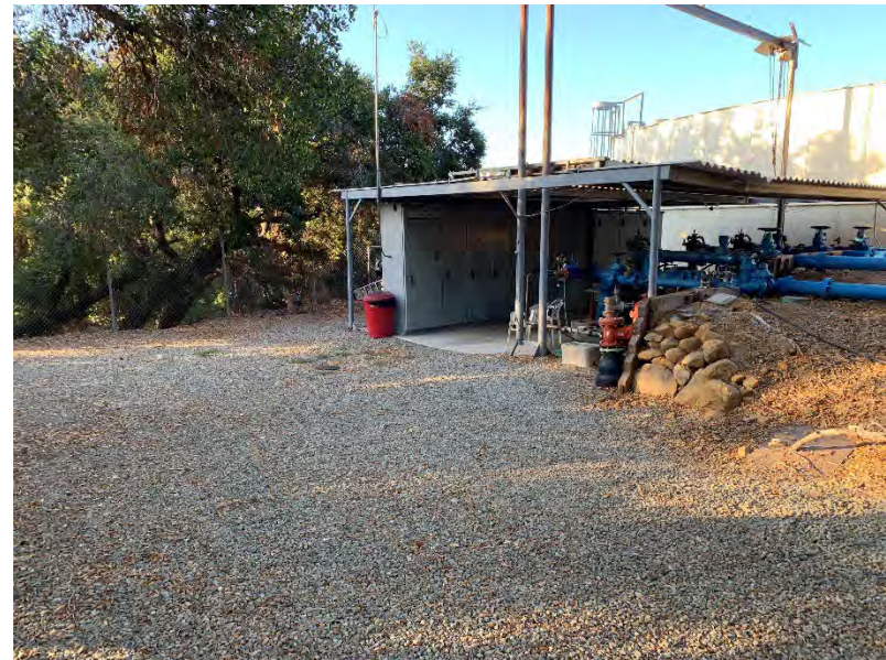
b. Parker pump station, existing tank in right background
