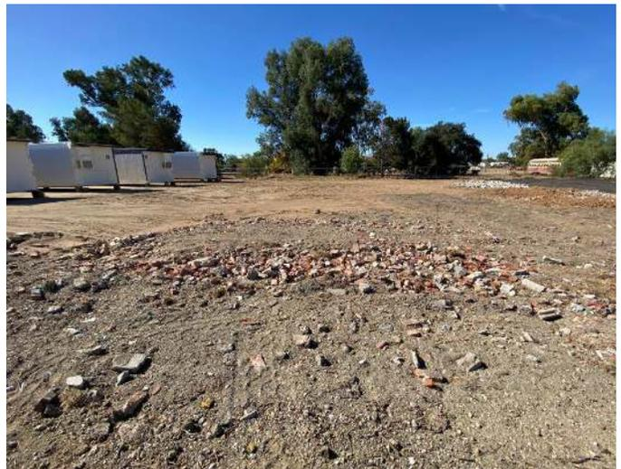
12. View of an area of imported brick, concrete, and stone observed in the central/eastern portion of the Site (presumably used as road-base), looking to the west.
